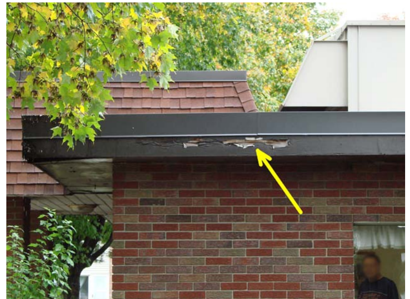
004_MI_1: Fascia detail - fascia needs repairs.
