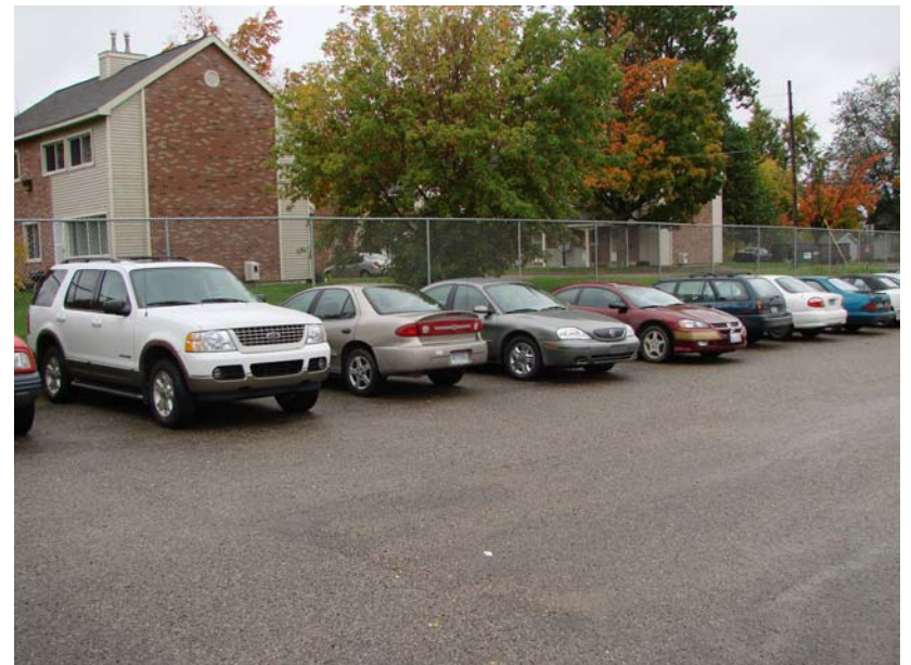
024_MI_1: Parking lot detail - asphalt paving needs to be sealed and striped.
