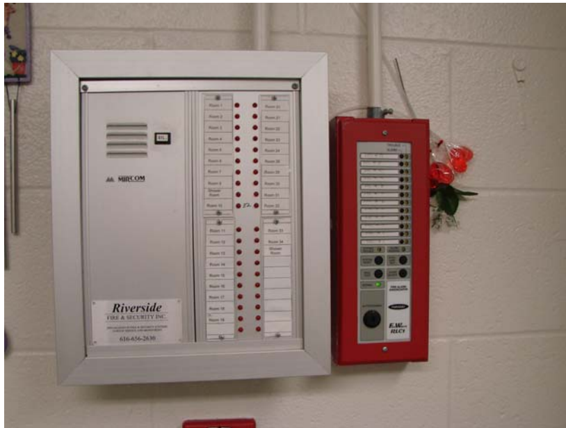
069_MI_1: Mircom nurse call, and Fire Watch fire alarm annunciator panels.
