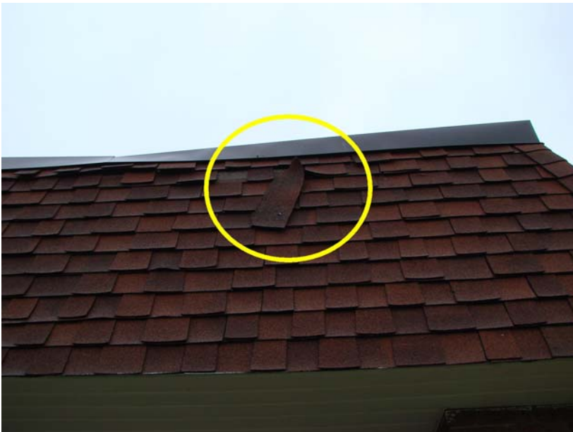
031_MI_1: Loose shingle at parapet wall above East Hall exit.
