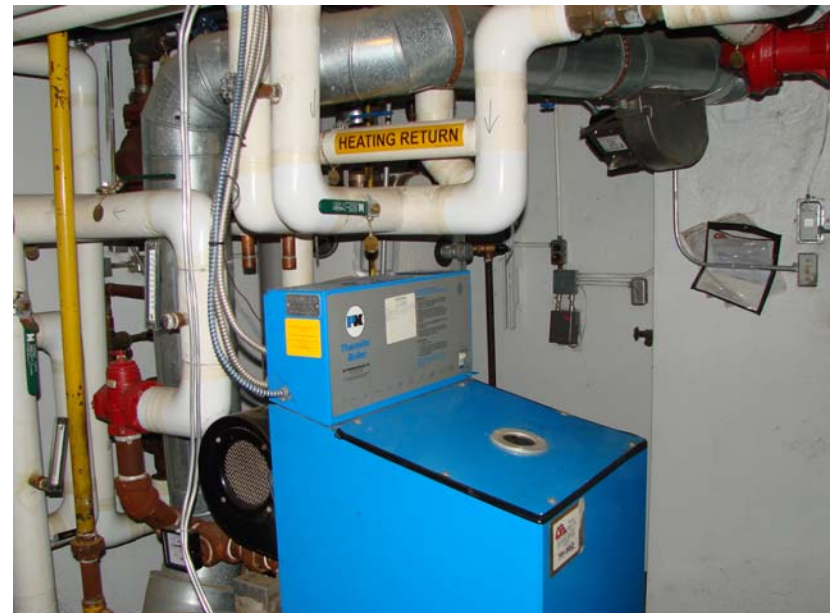
132_MI_1: South 2 Hall boiler room. Patterson-Kelly boiler, 700,000 BTUH (1998).
