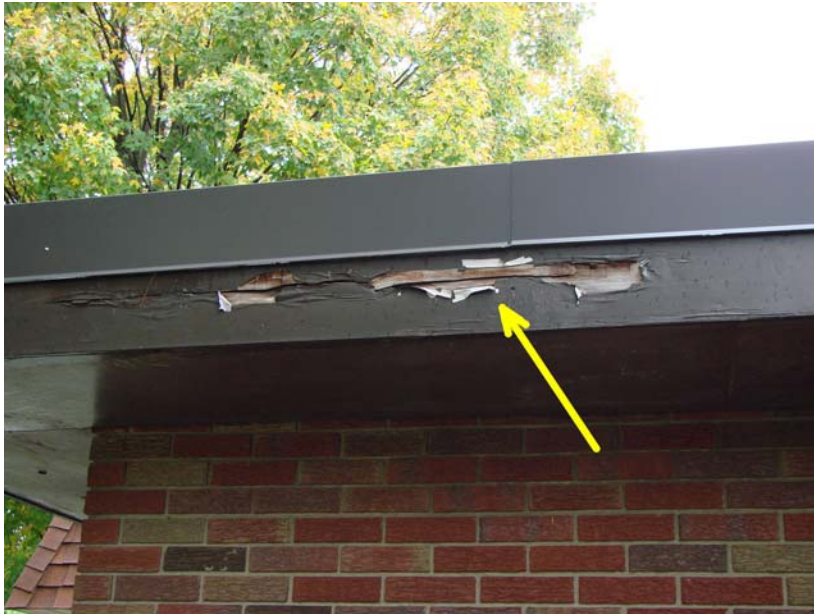
005_MI_1: Fascia detail - fascia needs repairs.
