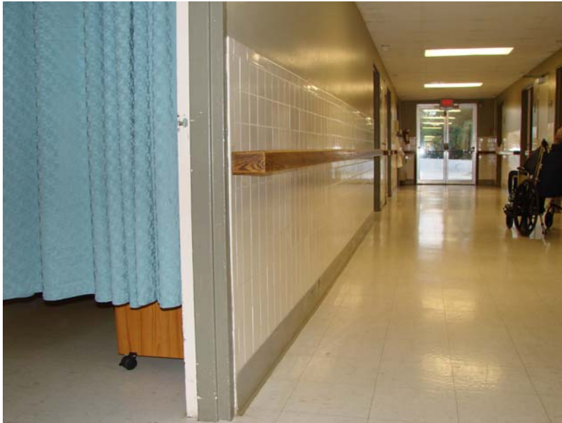
117_MI_1: South 2 Hall corridor detail - VCT floor, vinyl base, ceramic tile wainscot, wood handrail, painted wall (skim coat over CMU block wall), acoustic
