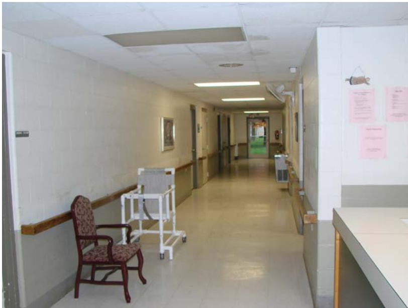
075_MI_1: South 1 Hall looking west from nurse station - note finishes include VCT floor, vinyl base, painted CMU block wall, wood handrail, acoustical grid
