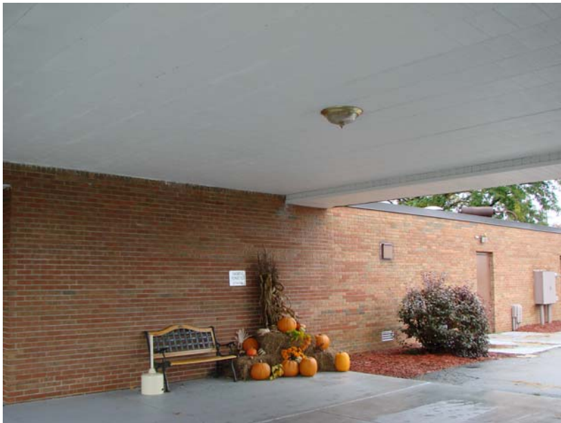
035_MI_1: Porte-cochere - pre-cast concrete planks with architectural -docks plank- finish.
