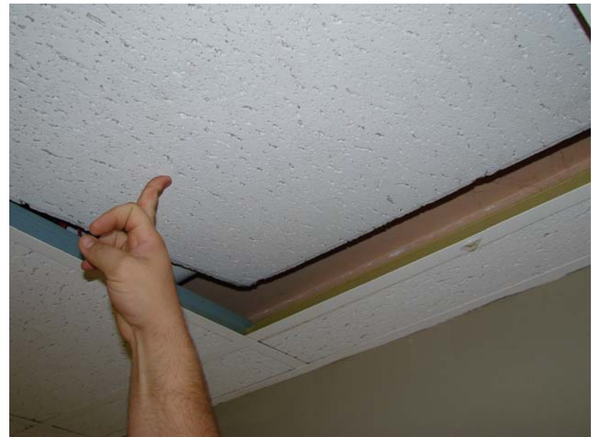
104_MI_1: Ceiling detail - minimal space above corridor ceiling grid.
