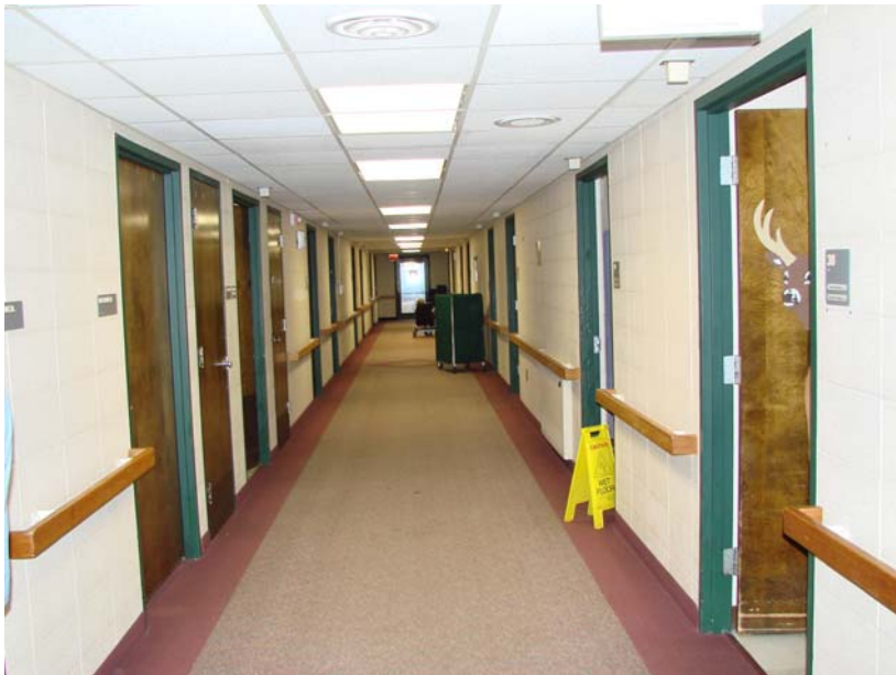
163_MI_1: West Hall looking south from nurse station - carpet, carpet base, painted CMU block walls, wood handrail, acoustical grid ceiling.
