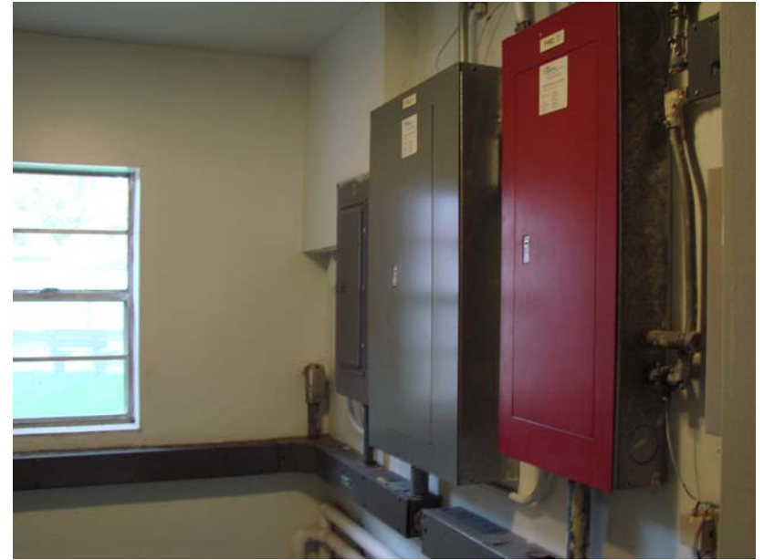
106_MI_1: Electrical sub-panels in South 2 Hall.
