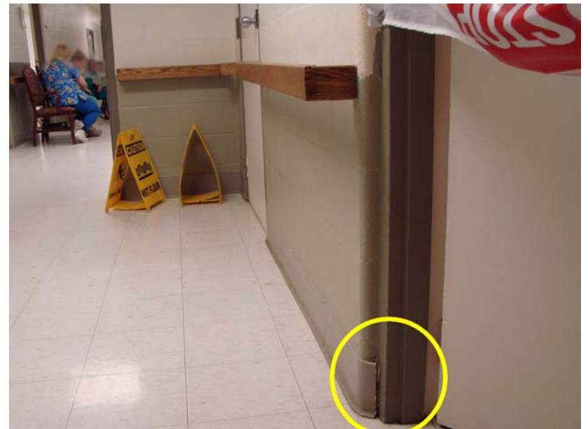
072_MI_1: Detail - wall base coming loose at door frame.
