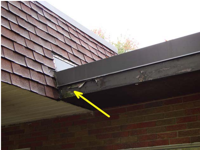
007_MI_1: Fascia detail - fascia needs repairs.
