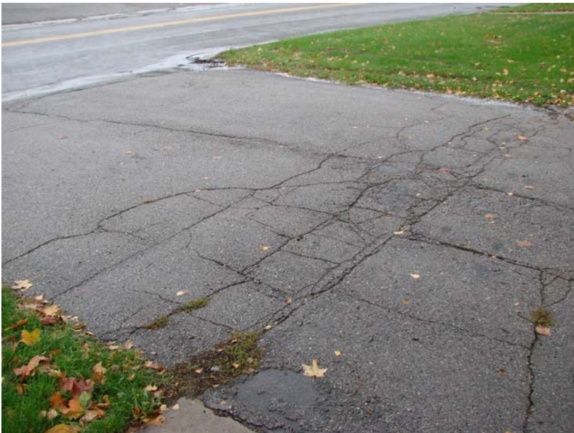
047_MI_1: Asphalt paving deterioration at service drive to dumpster on the south side of South 1 Hall.
