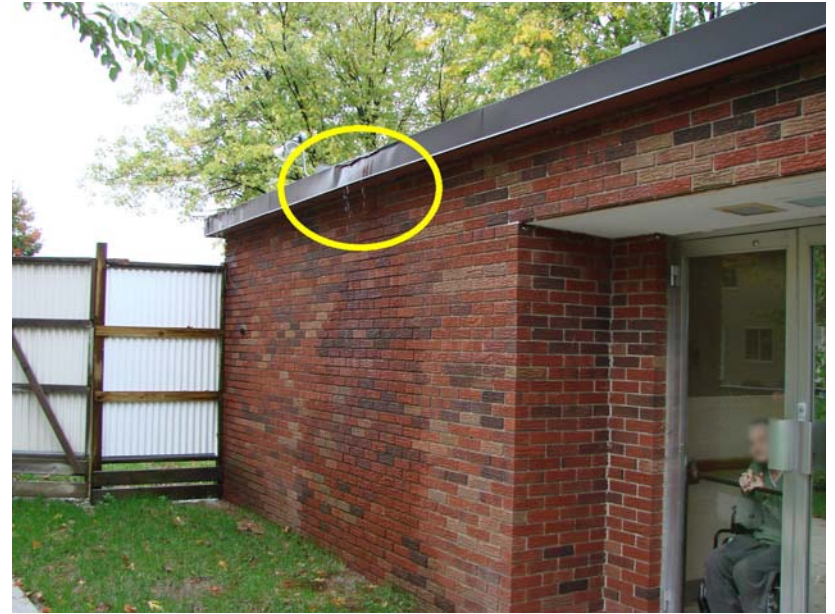
010_MI_1: Water running off edge of roof due to poor roof drainage.
