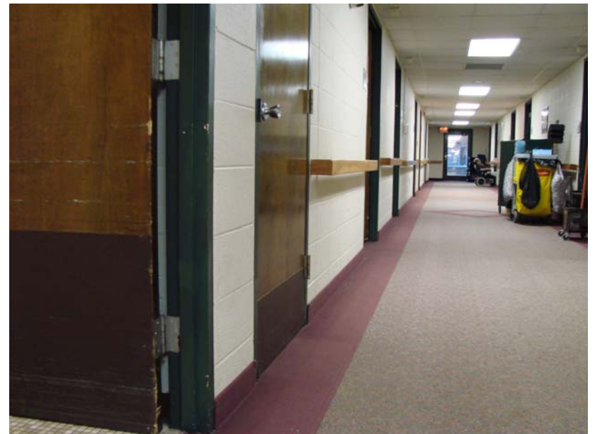
164_MI_1: Corridor detail - carpet, carpet base, painted CMU block walls, wood handrail, acoustical grid ceiling.
