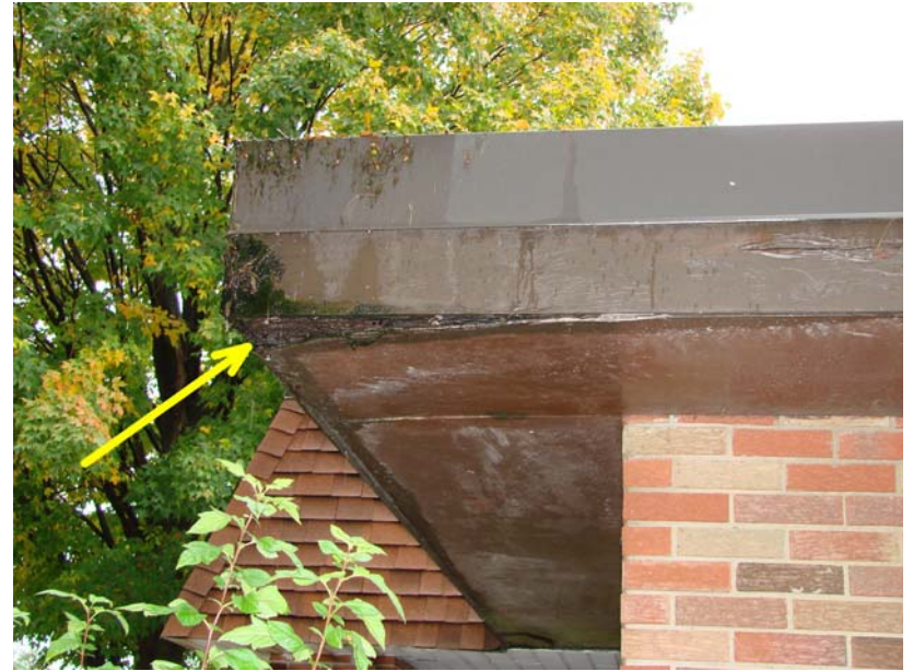
006_MI_1: Fascia detail - fascia needs repairs.
