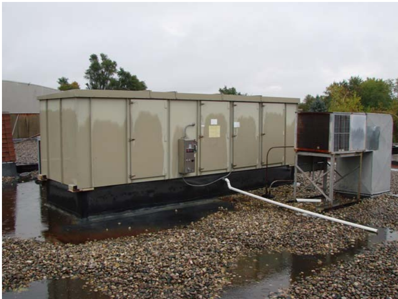
203_MI_1: Central Hall roof top air conditioner.
