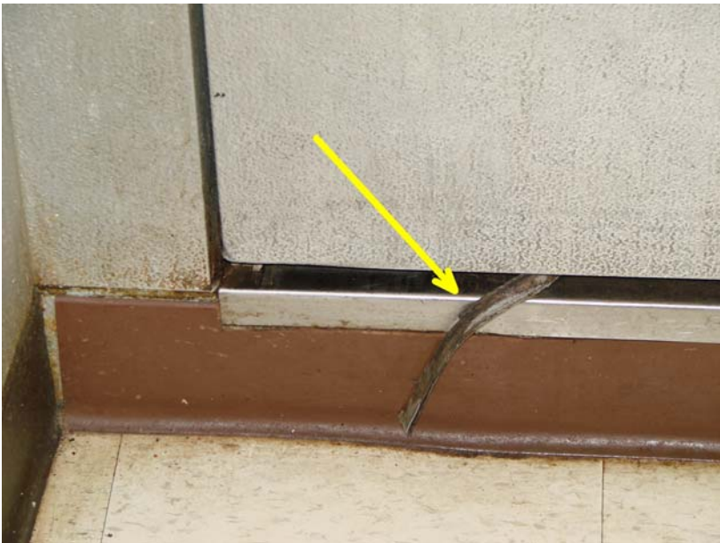
095_MI_1: Walk-in cooler door detail - loose seal.
