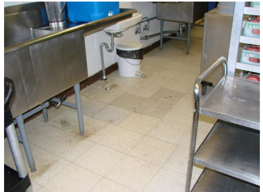
088_MI_1: Kitchen - VCT floor tile repairs.
