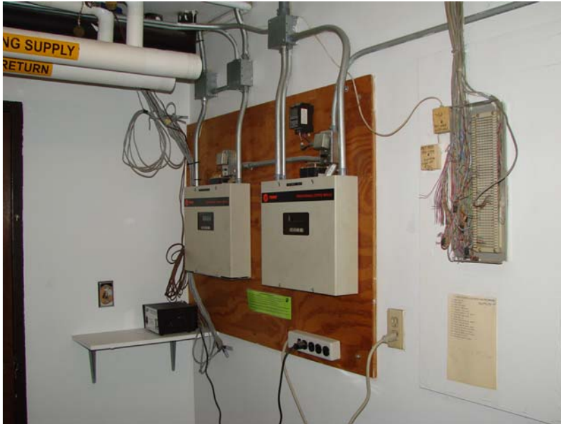
105_MI_1: Trane electronic HVAC controls.
