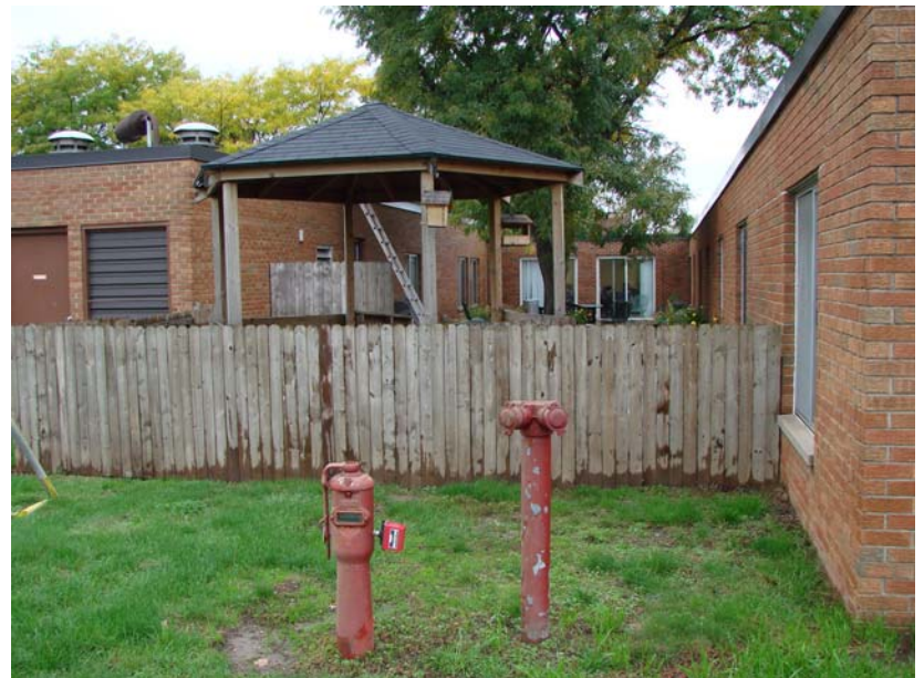
032_MI_1: Fire sprinkler connection, courtyard between Central Hall and East Hall.
