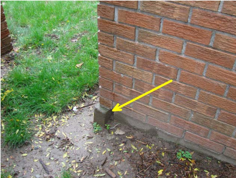
019_MI_1: Detail - curious foundation detail - concrete block protrusion.
