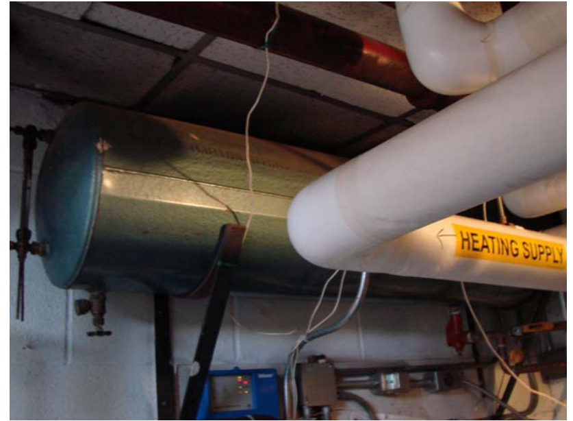
134_MI_1: Expansion tank (heating hot water).
