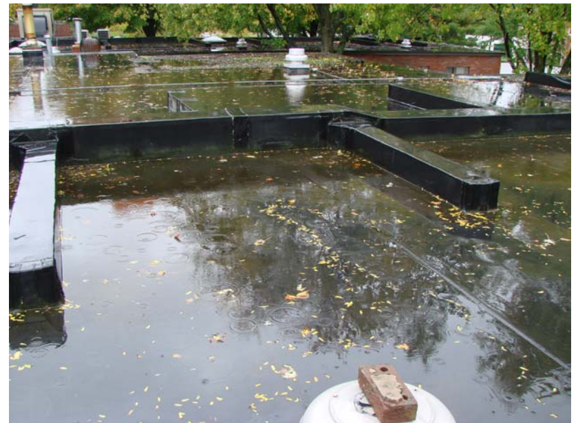
212_MI_1: Detail - HVAC ducts prevent proper roof drainage.
