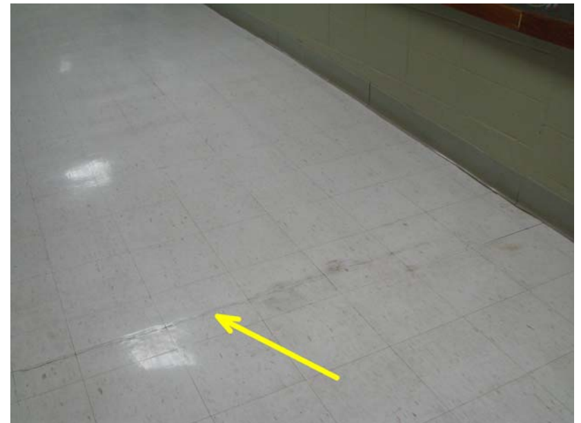
064_MI_1: VCT tile crack where corridor floor ramps out from South 1 Hall to center administrative hall.
