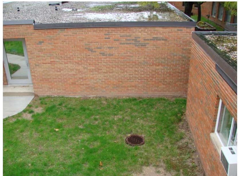
224_MI_1: Area drain at south end of West Hall.
