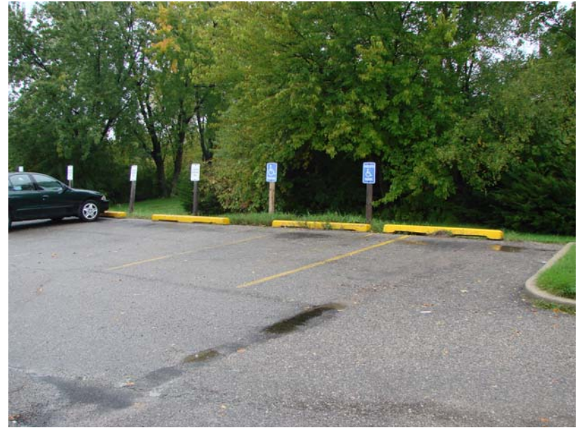
026_MI_1: Parking lot detail - asphalt paving needs to be sealed and striped.
