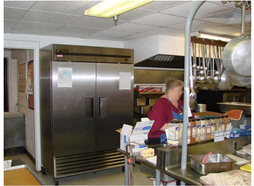
090_MI_1: Kitchen - True 2-door reach-in refrigerator.
