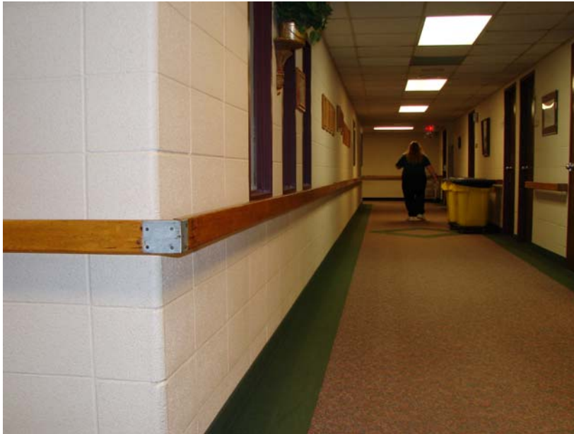
061_MI_1: Corridor detail, Administrative Hall, carpet, carpet base, painted CMU block wall, acoustical grid ceiling.
