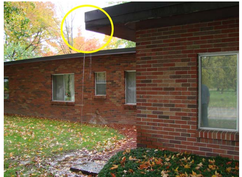
008_MI_1: Water running off edge of roof due to poor roof drainage.
