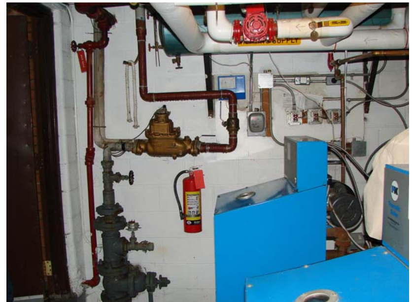
136_MI_1: Fire sprinkler riser (facility is only partially sprinkled).
