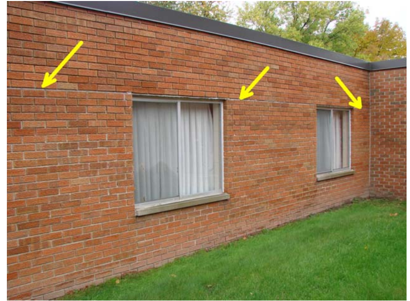
038_MI_1: Detail - mortar joint crack at brick lintel - runs length of North elevation of South 1 Hall.
