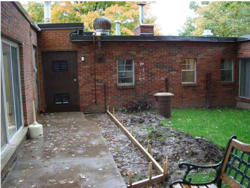
131_MI_1: Form boards - staff in widening sidewalk to boiler room.
