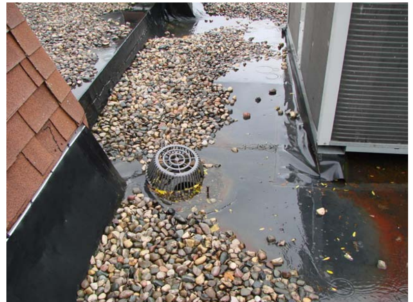
204_MI_1: Roof drain dislodged from its correct position.
