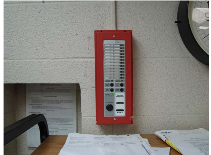
162_MI_1: Faraday fire alarm annunciator at nurse station.
