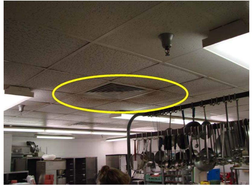
086_MI_1: Ceiling detail - dirty ceiling tile at air conditioner vent.
