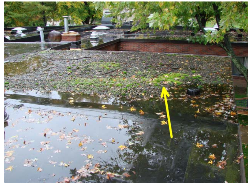
216_MI_1: Vegetation growing in roof ballast.
