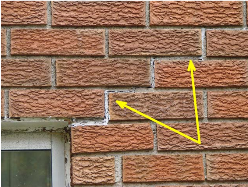
045_MI_1: Detail - mortar joint crack in South 2 Hall.
