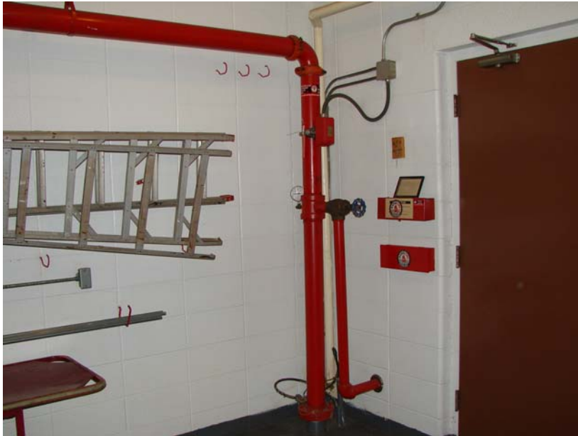
149_MI_1: Fire sprinkler riser for north wings (east & west) - note facility is not fully sprinkled.
