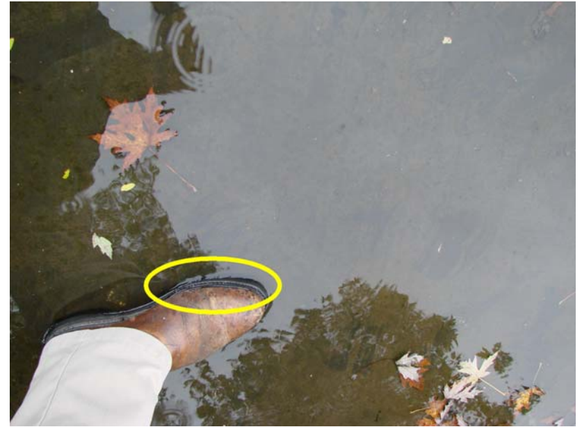
214_MI_1: Water ponding detail - approx 3-4- deep.
