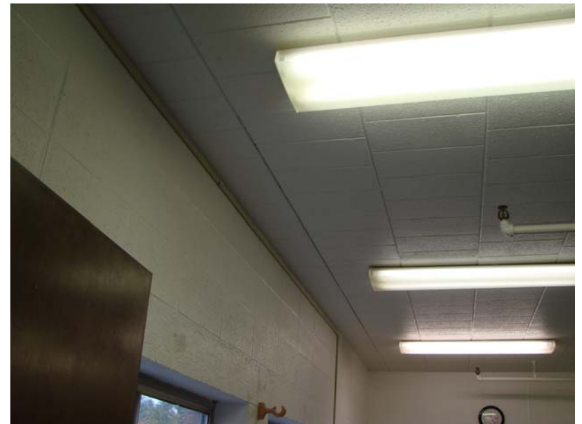
156_MI_1: Ceiling detail - painted, exposed pre-cast concrete ceiling planks with architectural -dock plank- finish.
