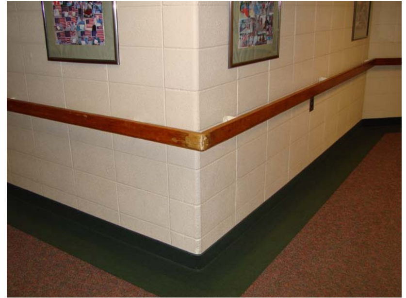
154_MI_1: Handrail detail - handrails need refinishing-better corner protection.
