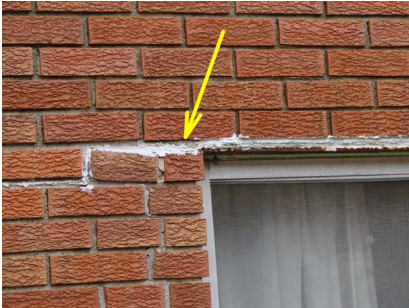
041_MI_1: Detail - mortar joint crack at brick lintel.
