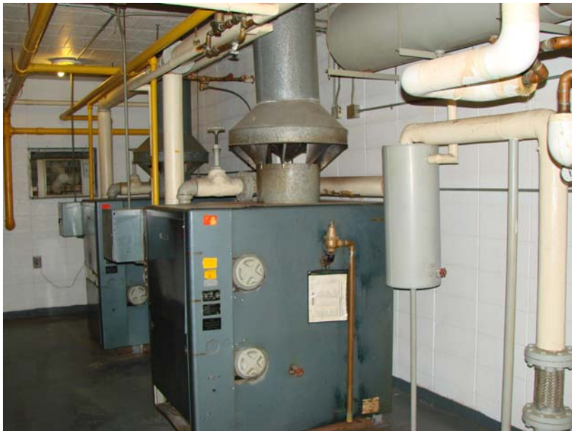
147_MI_1: Central wing boiler room - Weil-McClain boilers, 1,190,000 BTUH (20+ yrs).
