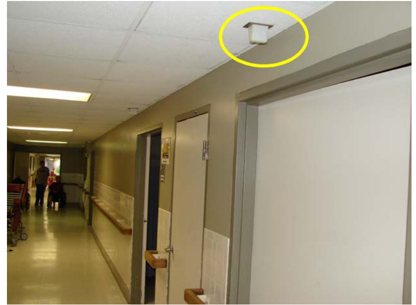
118_MI_1: South 2 corridor detail - nurse call lights in ceiling.
