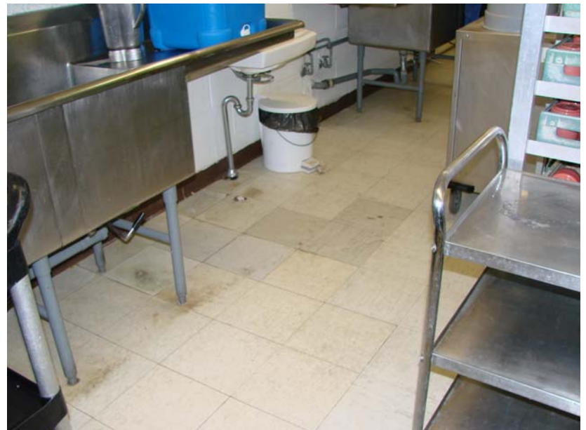
088_MI_1: Kitchen - VCT floor tile repairs.
