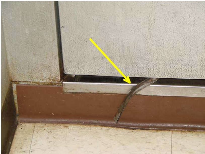
095_MI_1: Walk-in cooler door detail - loose seal.
