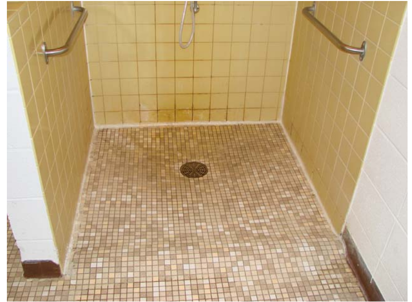
190_MI_1: Shower floor detail - average condition.
