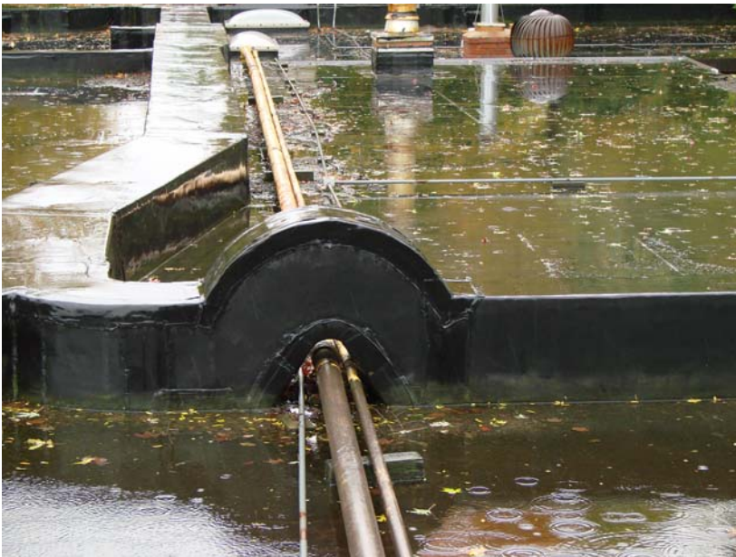
219_MI_1: South Hall 1 detail - HVAC duct arched over conduit pipe.
