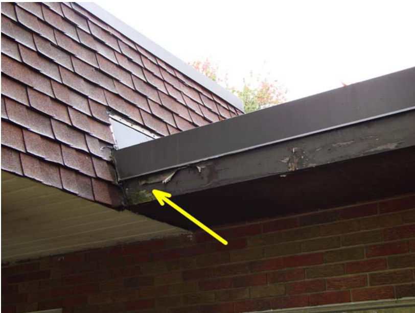
007_MI_1: Fascia detail - fascia needs repairs.
