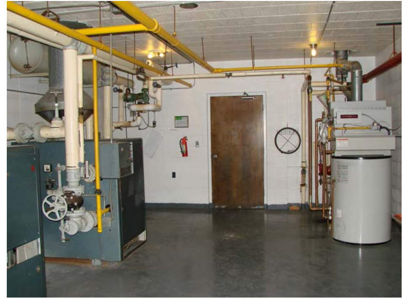
146_MI_1: Central corridor boiler room - Weil-McClain boilers, Lochinvar water heaters.
