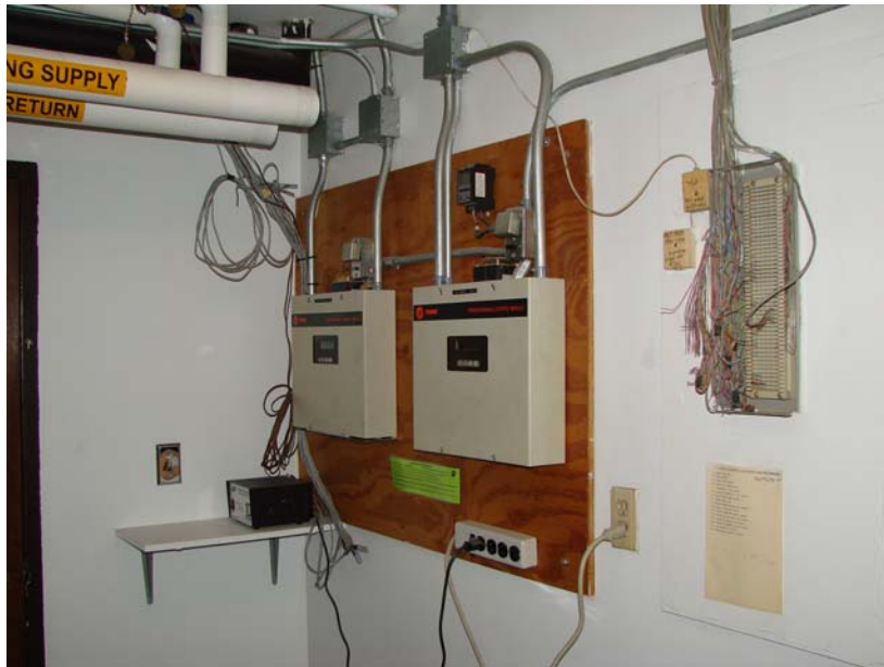
105_MI_1: Trane electronic HVAC controls.
