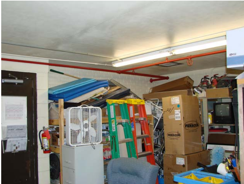
065_MI_1: Fire sprinklers in maintenance office. Note facility is only partially sprinkled.
