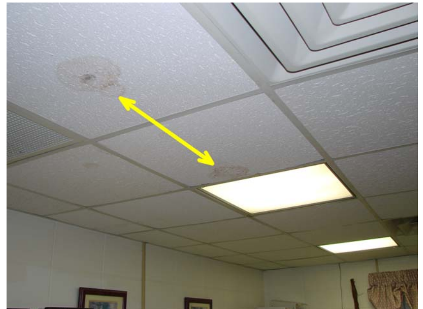
200_MI_1: Water stains on ceiling tile in therapy office.
