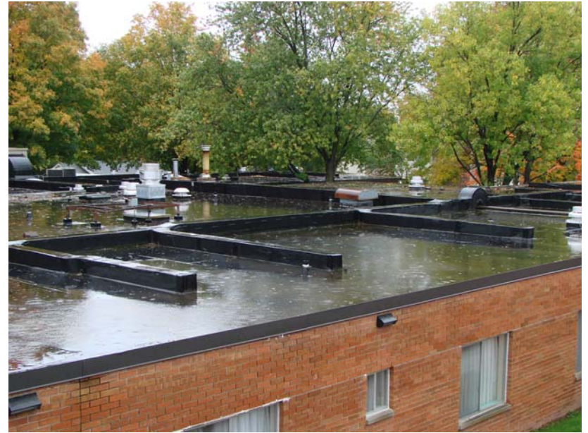
210_MI_1: South Hall 1 roof - note EPDM rubber roof membrane is applied over corridor HVAC ducts.
