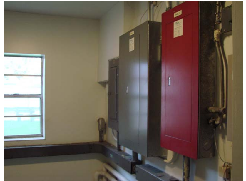
106_MI_1: Electrical sub-panels in South 2 Hall.
