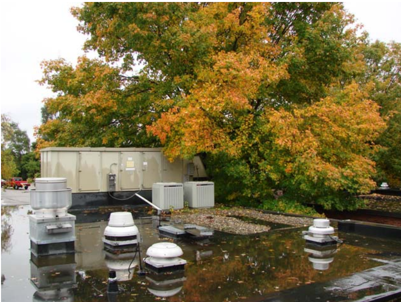
215_MI_1: Tree growing between South 1 and South 2 Halls needs to be trimmed away from air conditioners.
