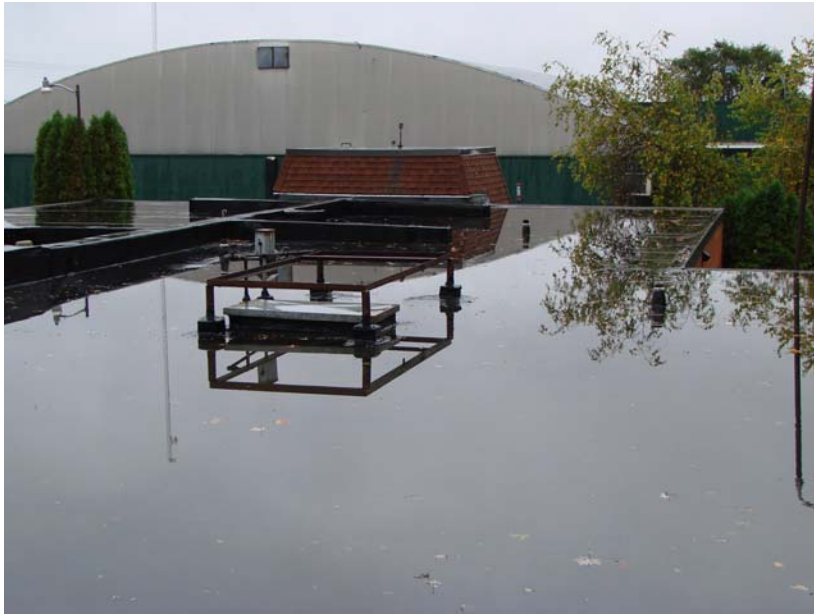
209_MI_1: Water ponding on South Hall 1 roof - drainage obstructed by HVAC ducts.
