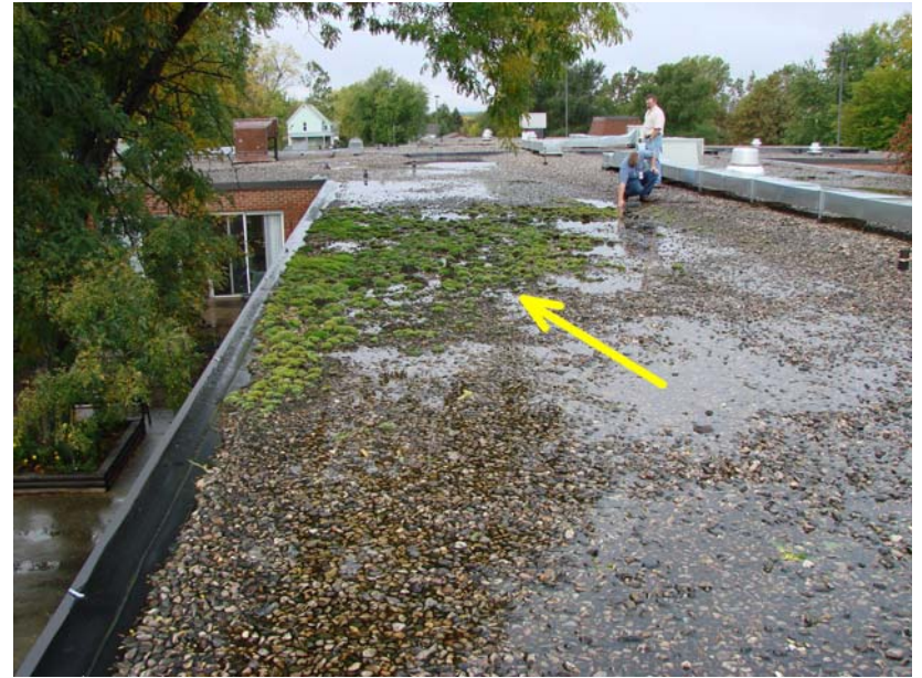
230_MI_1: Vegetation growing in roof ballast.
