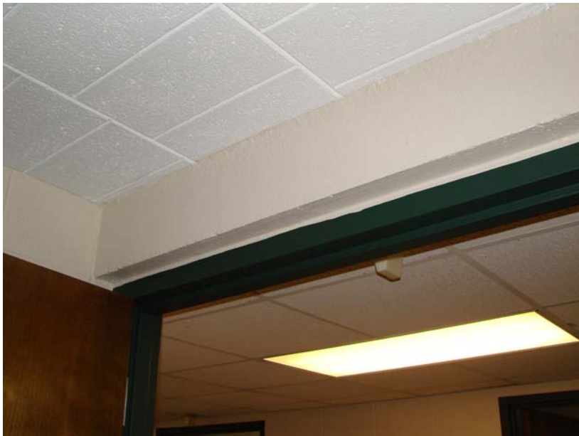
179_MI_1: Ceiling detail - exposed concrete plank ceiling in resident rooms, dropped acoustical grid ceiling in corridor.
