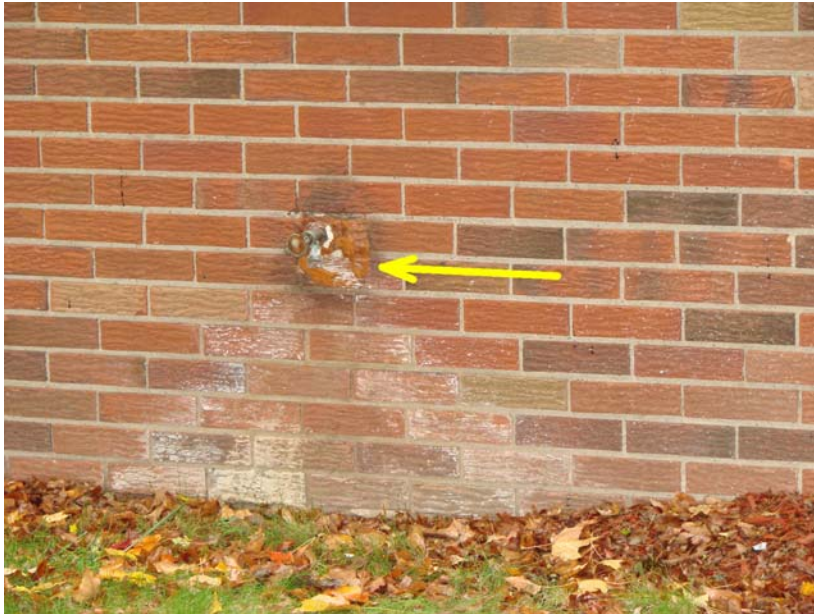
009_MI_1: Water faucet - insulation needs to be monitored for deterioration and maintained.
