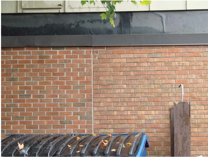
049_MI_1: Detail - expansion joint at kitchen addition.
