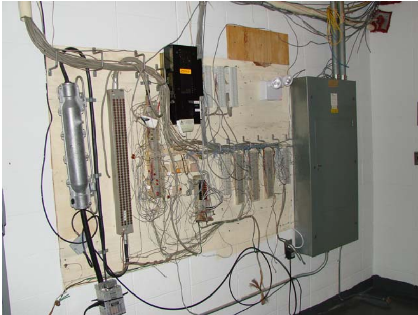
141_MI_1: Telephone patch panels.
