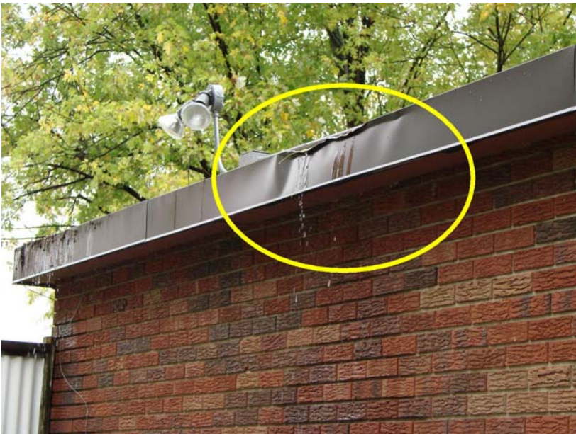
011_MI_1: Water running off edge of roof due to poor roof drainage.
