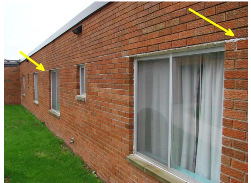
016_MI_1: Detail - mortar joint crack at brick lintel - runs length of west elevation of West Hall.
