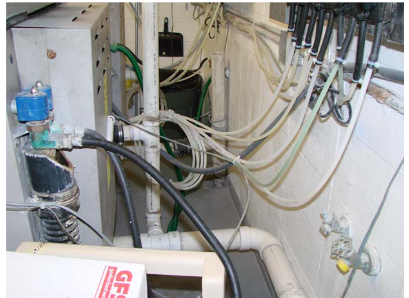
144_MI_1: Laundry - washer drain connection.
