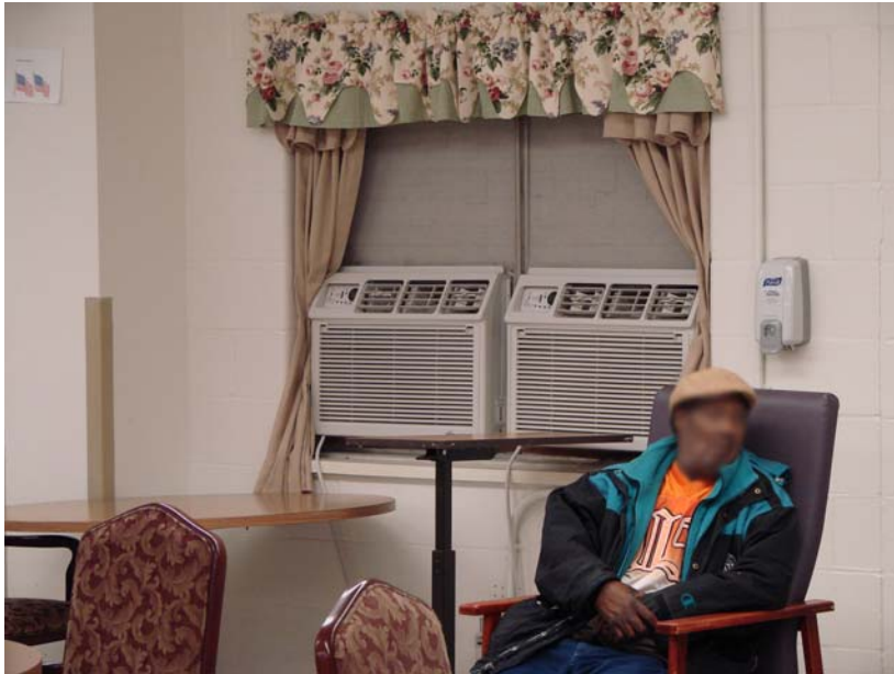
077_MI_1: Window unit air conditioners in South 1 dining room.
