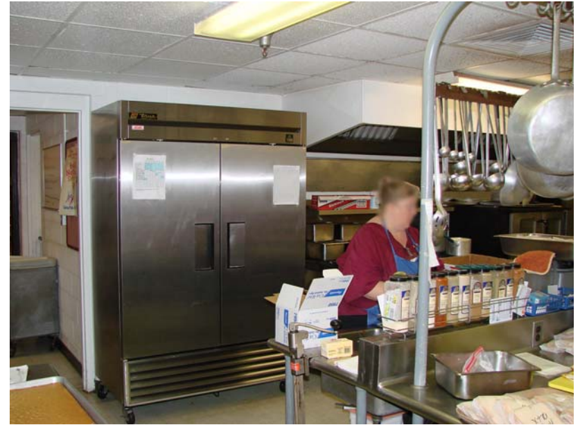
090_MI_1: Kitchen - True 2-door reach-in refrigerator.
