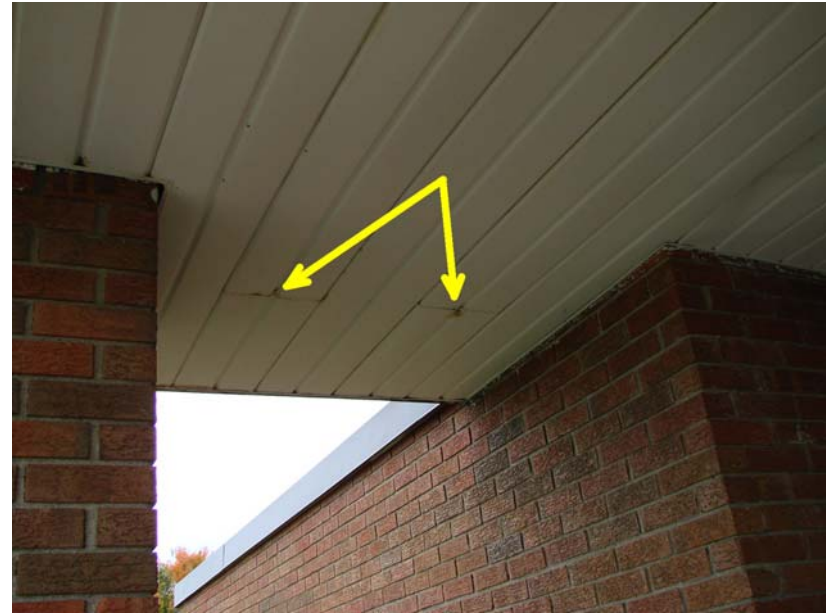
030_MI_1: Rust stains at East Hall exit awning ceiling.
