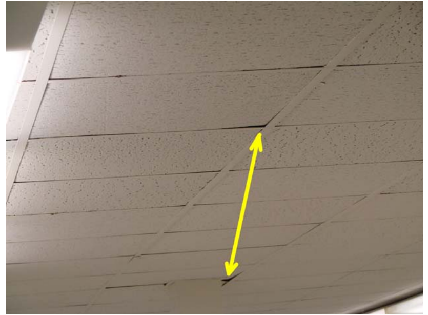
078_MI_1: Dining room ceiling detail - tiles are warping at corners.
