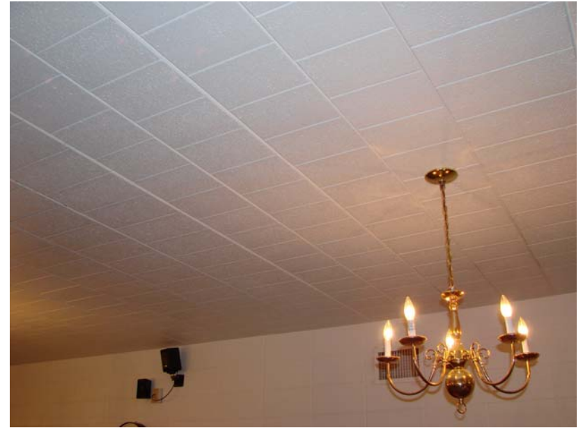
058_MI_1: Ceiling detail - pre-cast concrete plank ceiling with architectural -dock plank- finish.
