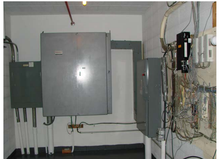
140_MI_1: Electrical room - 600 Amp main service, telephone patch panels.
