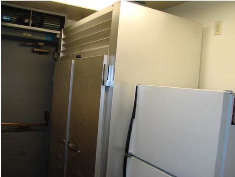
022 P_W: Kitchen - residential refrigerator, Traulsen 2-door freezer. (Note - freezer compressor was replaced 5-2-07).
