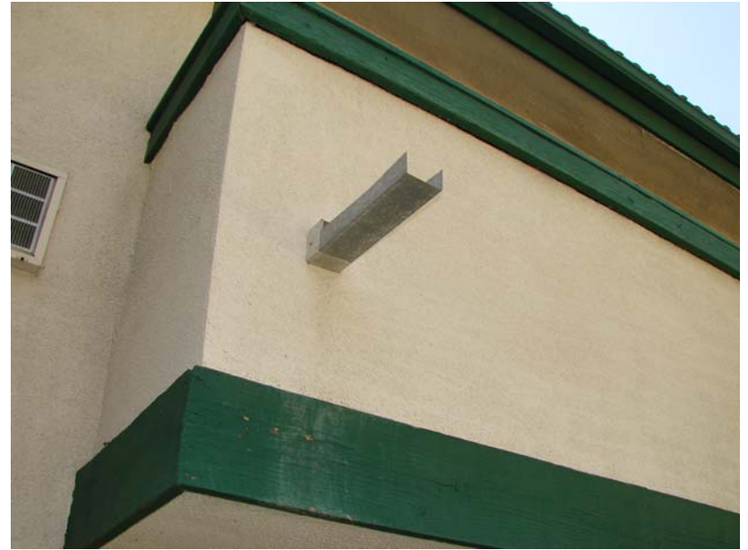
179 P_E: Balcony drain scupper with extension.
