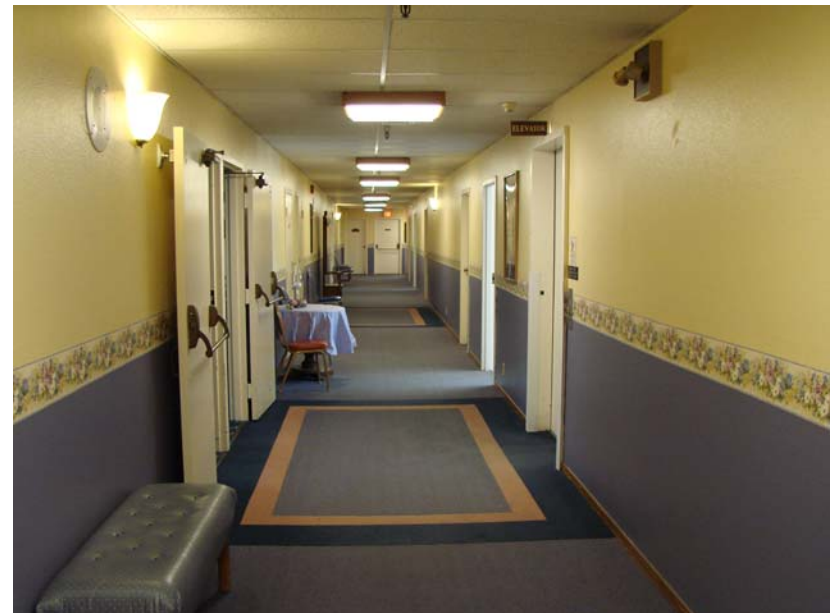
093 P_E: Palm East - typical 2nd floor corridor. Wood base, painted walls, no handrails, wallpaper border transition. Paint and border are currently being
