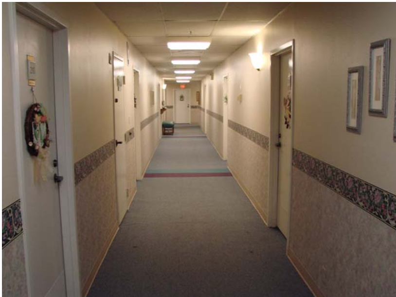
044 P_W: Typical 2nd floor corridor - note carpet, rubber base, wallpaper below border, paint above.
