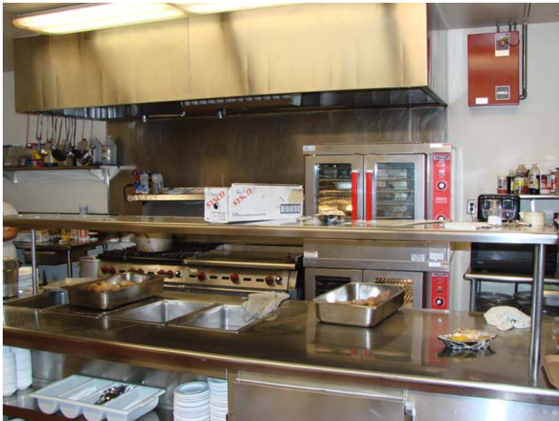
072 P_E: Kitchen - Wolf 6-burner stove with double oven & griddle; Vulcan convection ovens (2).
