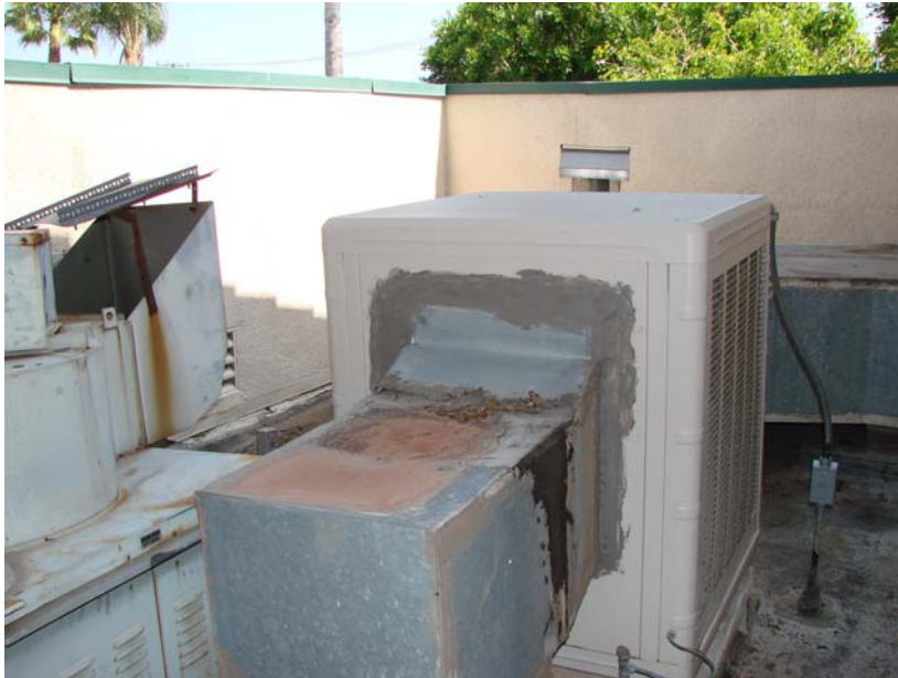
054 P_W: Kitchen swamp cooler in roof well.
