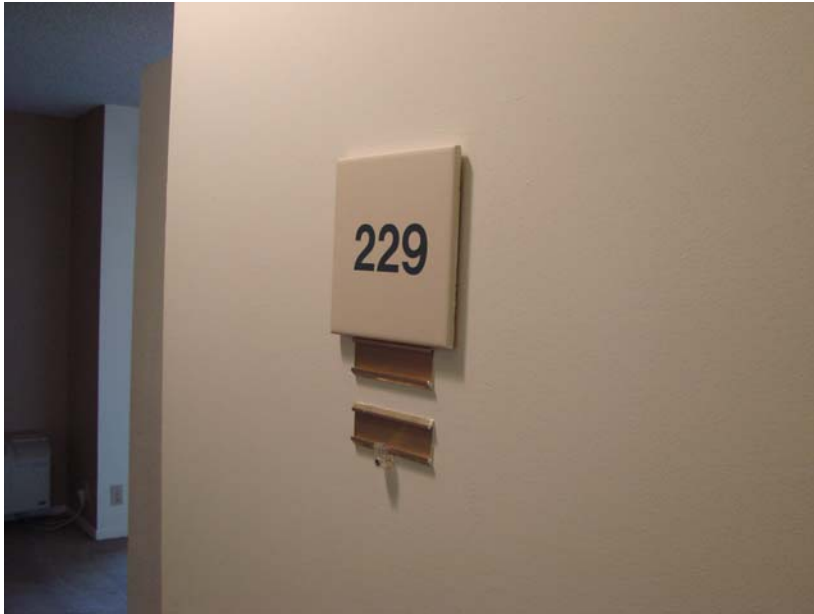
126 P_E: Typical room signage.
