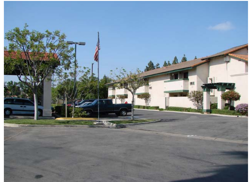
013 P_E: West elevation of Palm East (looking north).
