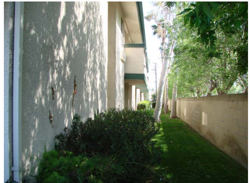
077 P_W: Palm West west elevation looking south.
