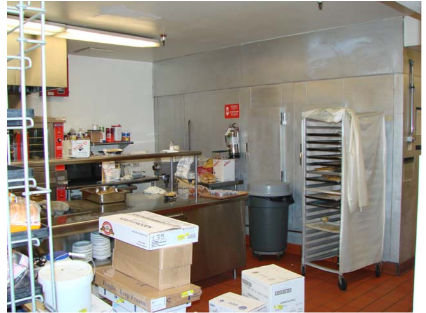
071 P_E: Kitchen - walk-in freezer-cooler.
