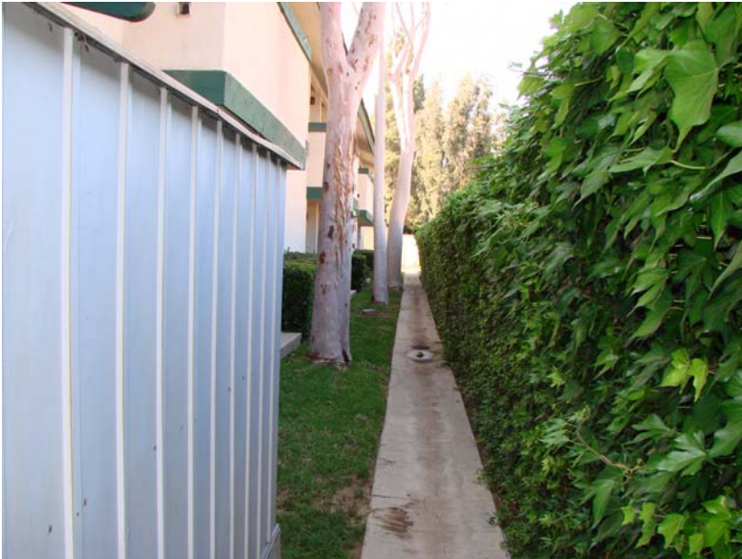
040 P_E: Palm East east elevation looking north.
