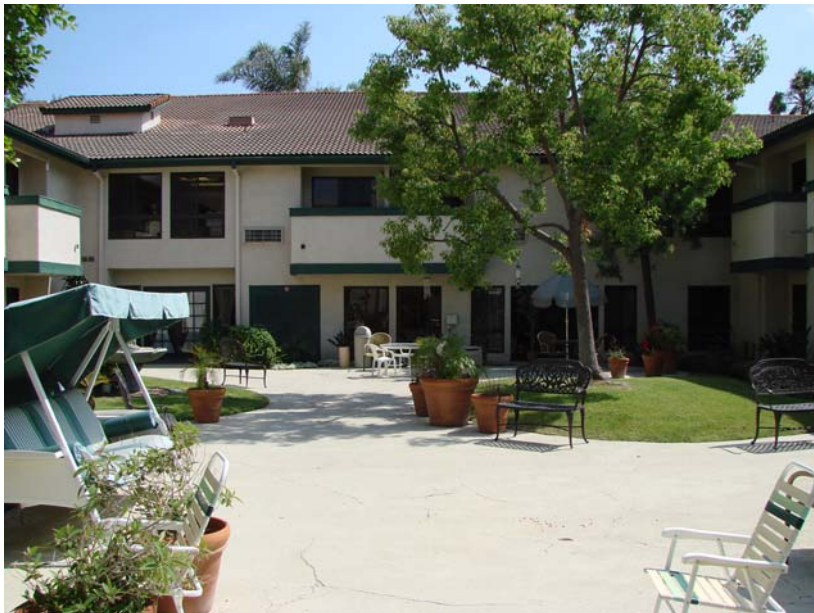
156 P_E: Interior courtyard.
