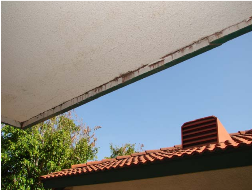
070 P_W: Rotten wood trim on 2nd floor balcony - water penetration behind wood.
