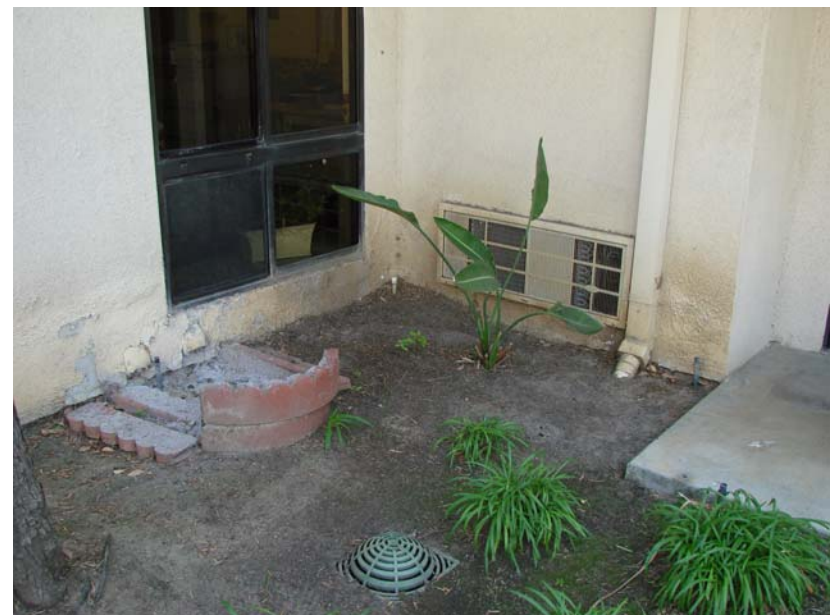
173 P_E: Laundry dryer vents - consider adding a wire cage lint trap.
