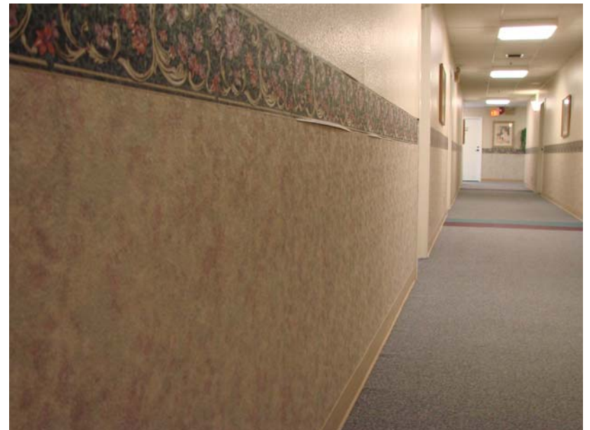
037 P_W: Detail - West Hall - wall covering below border, paint above.
