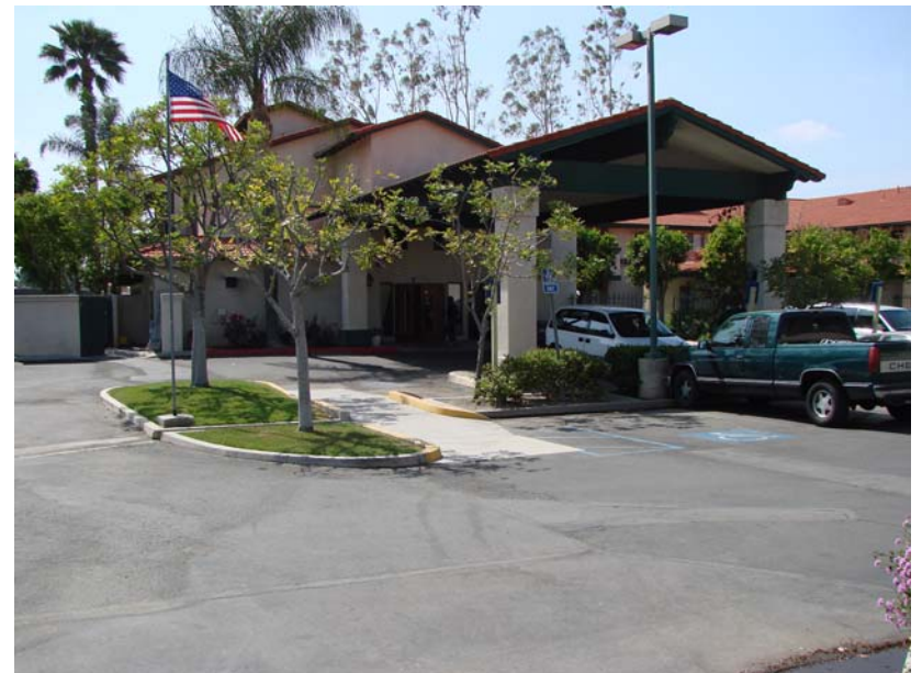
005 P_W: Palm West front (east) elevation;, main entrance.
