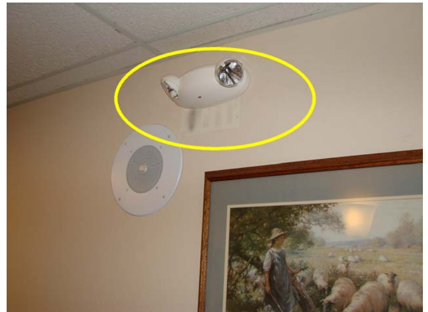
085 P_E: New emergency light. Note paint mark from original light outline.
