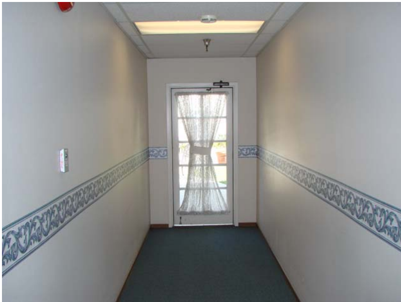
084 P_E: West Hall alcove leading to interior courtyard.
