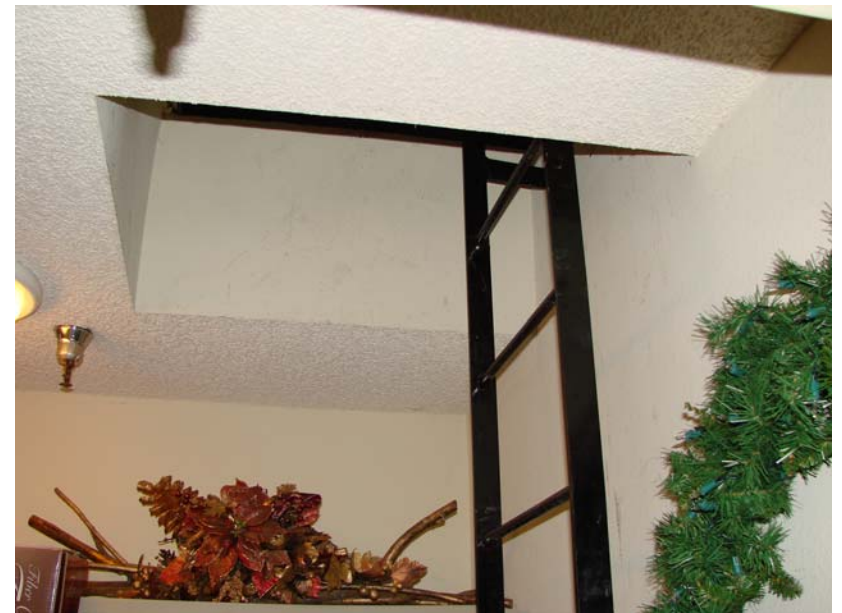
121 P_E: Ships' ladder in storage closet to roof well.
