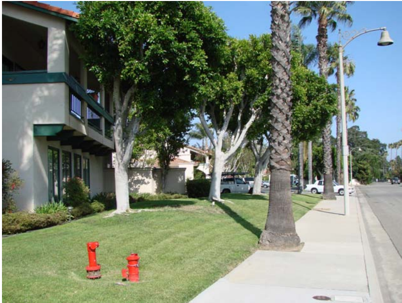
098 P_W: Southwest property line looking east along road frontage. Fire stand pipe.
