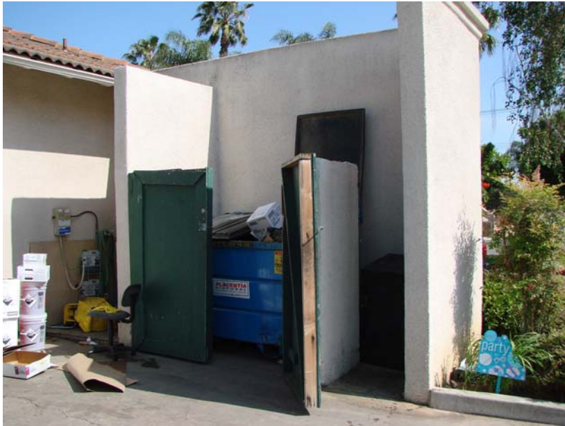
018 P_E: Trash dumpster at service area.
