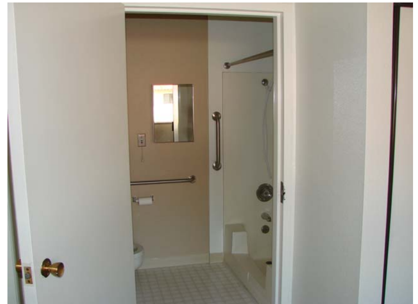
133 P_E: Typical resident unit. Remodel in process between residents.
