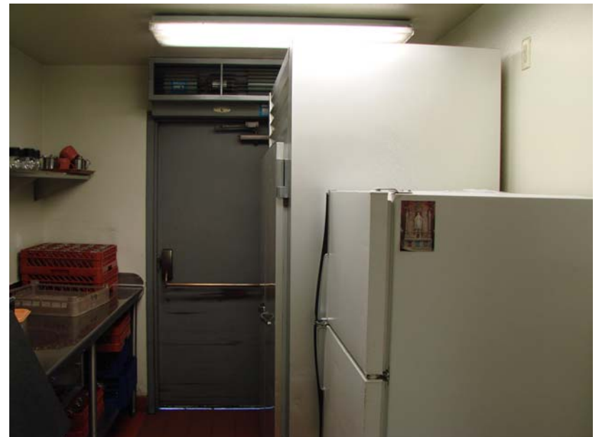
021 P_W: Kitchen - residential refrigerator, Traulsen 2-door freezer. (Note - freezer compressor was replaced 5-2-07).
