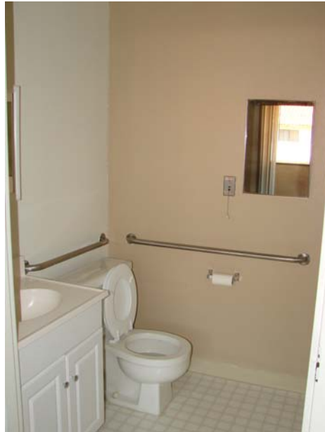
134 P_E: Typical resident unit. Remodel in process between residents.
