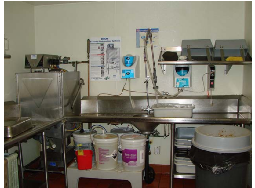
075 P_E: Kitchen - dishwashing area.
