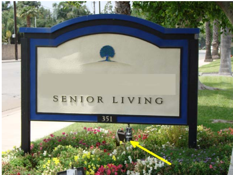
002 P_E: Facility identification sign. Note broken sign lighting.
