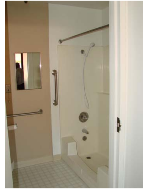
135 P_E: Typical resident unit. Remodel in process between residents.
