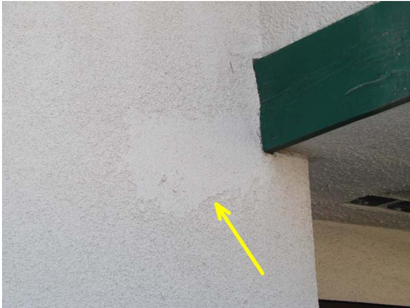
046 P_E: Wall patch on east elevation at balcony.
