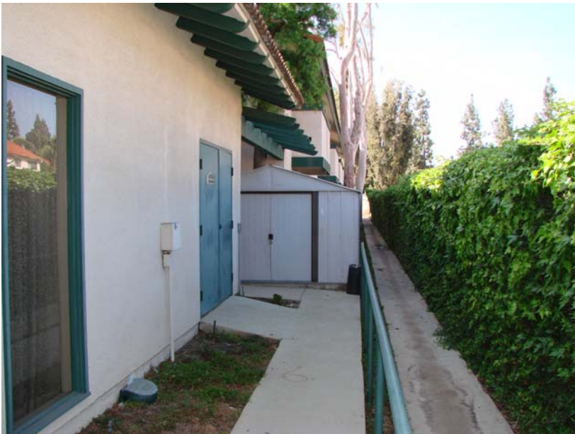
036 P_E: Palm East east elevation looking north. Storage building and main electrical closet at stair well #3.
