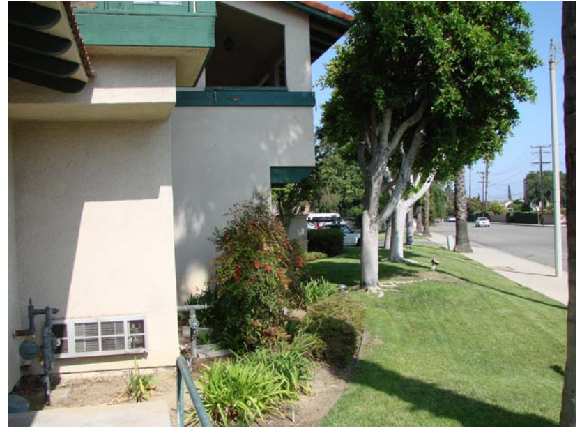
087 P_W: Southwest property line looking east along road frontage.
