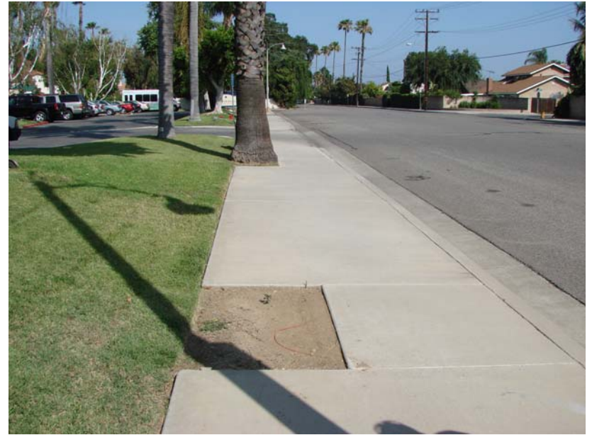
099 P_W: Removed palm tree in public right of way - consider petitioning City to replace tree or fill in with concrete.
