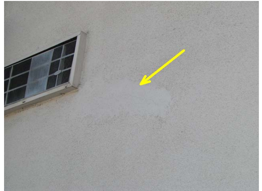
045 P_E: Wall patch on east elevation at PTAC unit.
