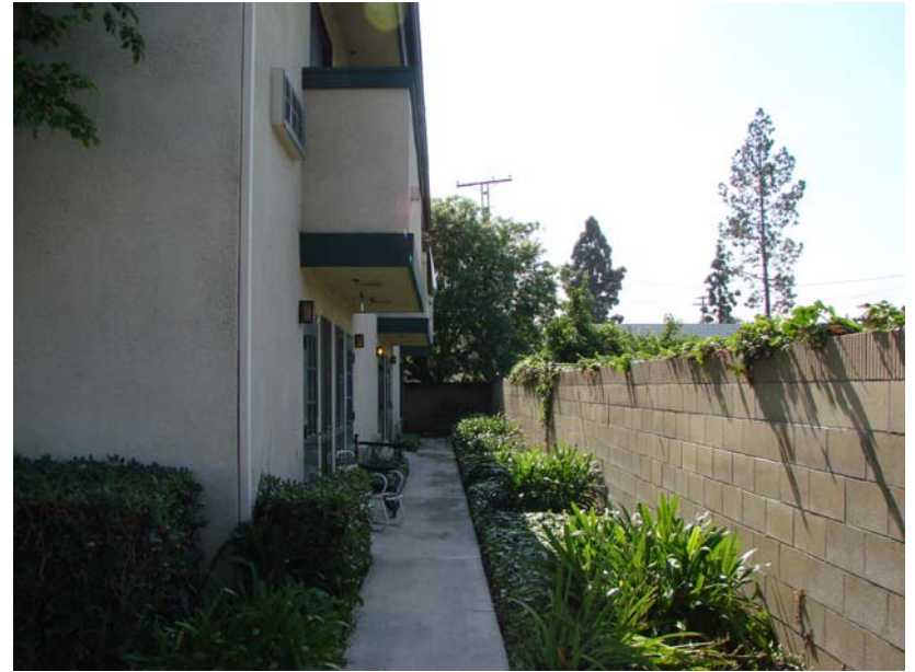
075 P_W: North elevation of Palm West looking west.
