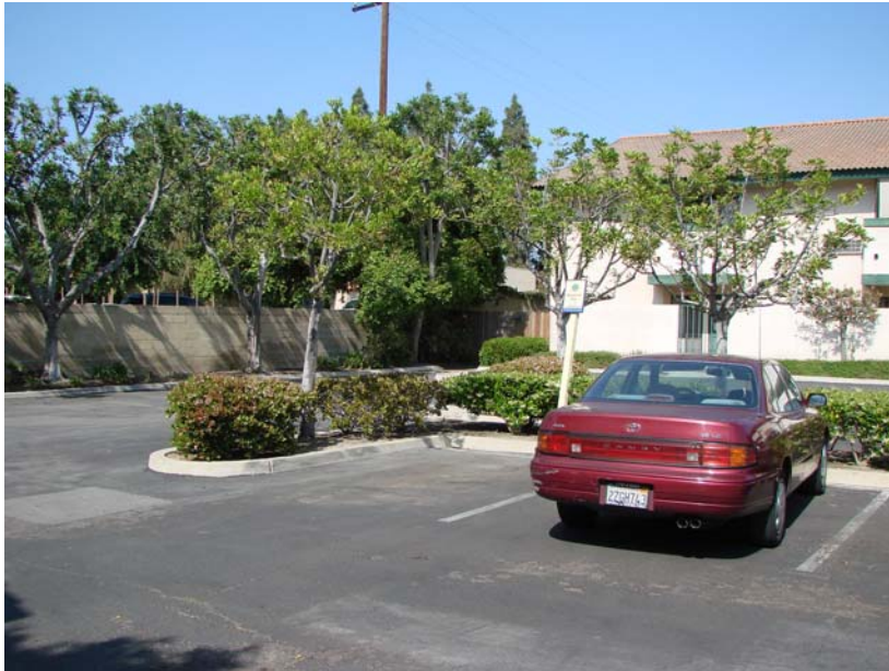
074 P_W: Parking between buildings - northwest elevation of Palm East.
