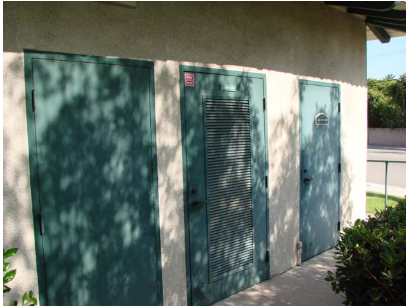
082 P_W: Electrical closet & elevator equipment rooms.
