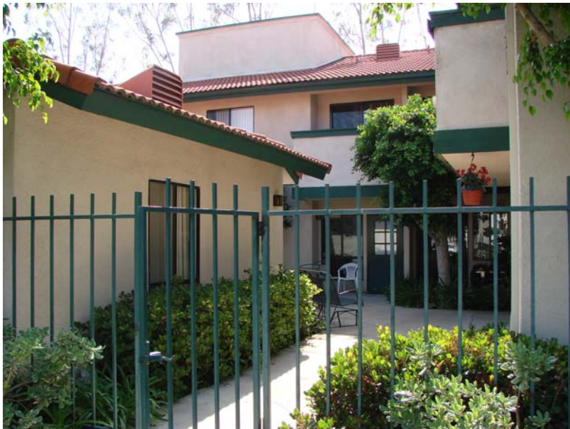
068 P_W: Palm West north courtyard.
