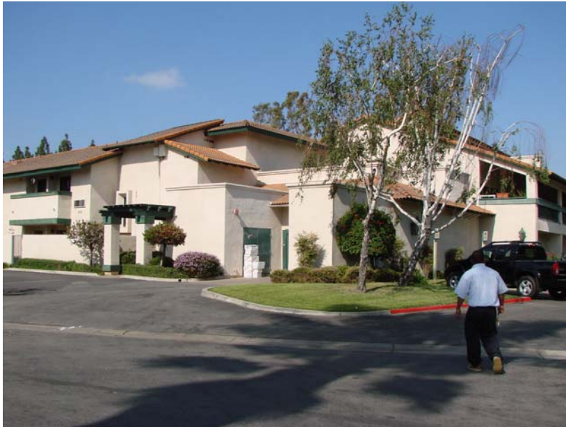
014 P_E: Palm East service entrance - water heater room & kitchen delivery area.
