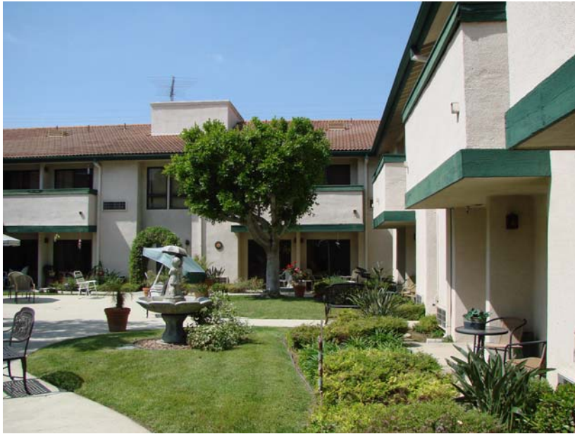
158 P_E: Interior courtyard.
