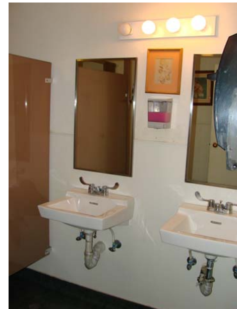
097 P_E: Palm East - 2nd floor public restroom.
