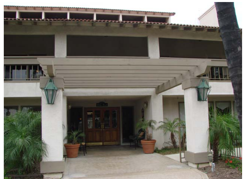
04-2009-04-23_DSC09261: After - repaired and re-painted wood.
