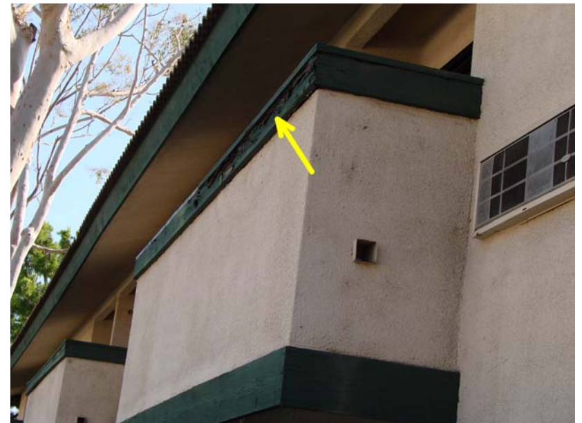
12-2007-05-02_042 P_E: Before - Detail - rotten trim on 2nd floor balcony.
