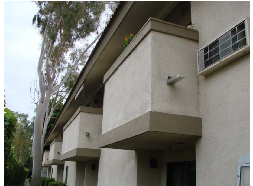
14-2009-04-23_DSC09246: After - repaired and re-painted wood.
