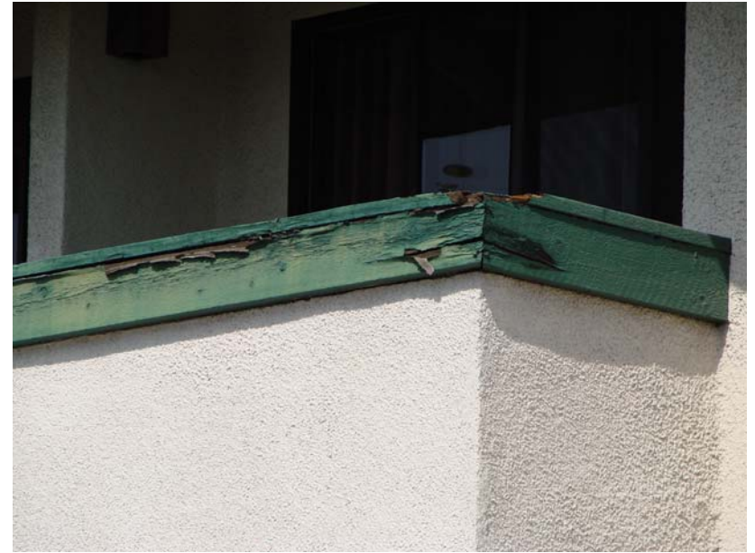
10-2007-05-02_034 P_E: Before - Detail - rotten wood trim on 2nd floor balconies.
