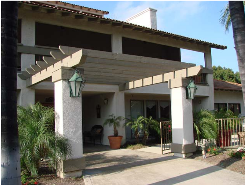
05-2009-04-23_DSC09433: After - repaired and re-painted wood.
