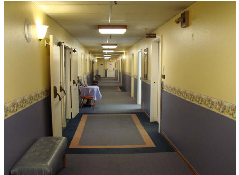
22-2007-05-02_093 P_E: Before - Palm East - typical 2nd floor corridor. Wood base, painted walls, no handrails, wallpaper border transition. Paint and border are
