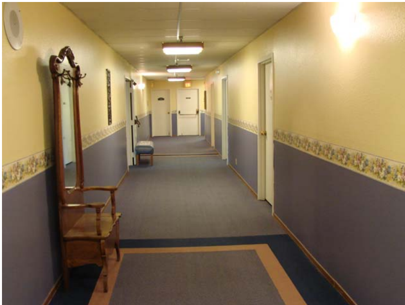
23-2008-05-19_DSC08586: Before - Palm East - typical 2nd floor corridor. Wood base, painted walls, no handrails, wallpaper border transition. Paint and
