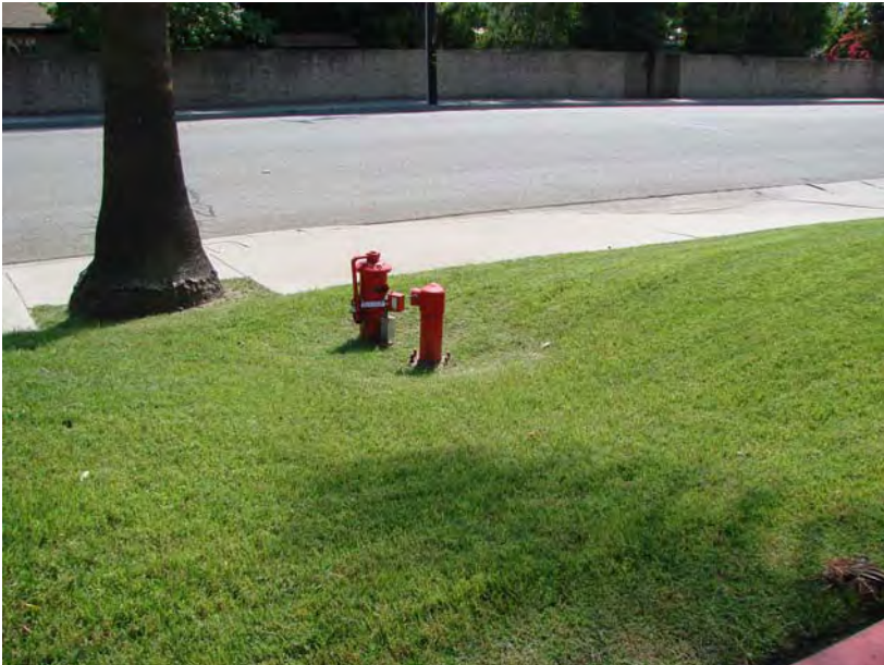
012 P_E: Fire sprinkler stand pipe.
