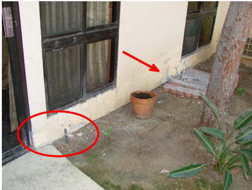
170 P_E: Courtyard detail - water damage outside private dining room (possibly from sprinklers-).
