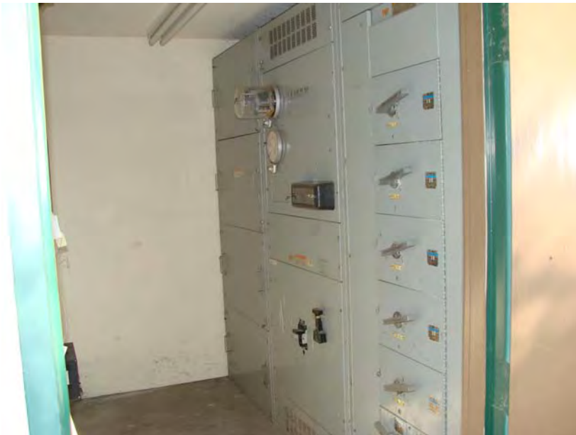
084 P_W: Main electric service - 1000 Amp main panel.
