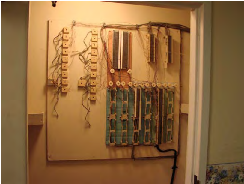
116 P_E: 2nd Floor West Hall electrical closet; telephone patch panel.
