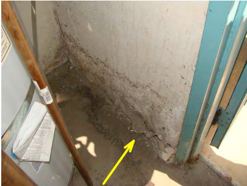
030 P_E: Water damage in water heater closet.
