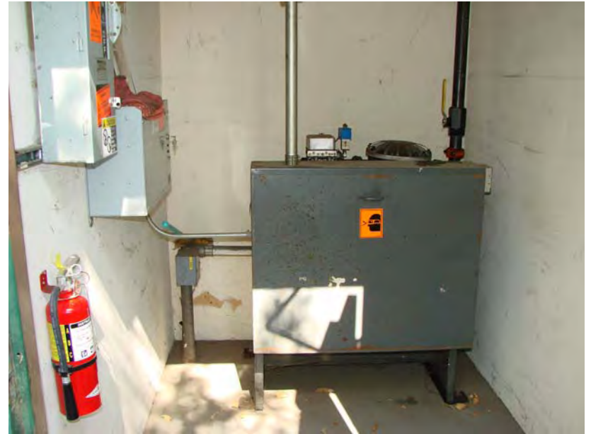
083 P_W: Hydraulic elevator equipment room.
