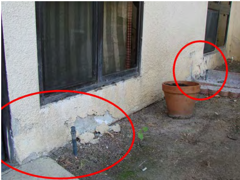
172 P_E: Courtyard detail - water damage outside private dining room (possibly from sprinklers-).
