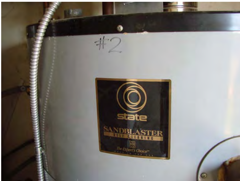
092 P_W: State water heater (#2), 100-gal, 260,000 BTUH.
