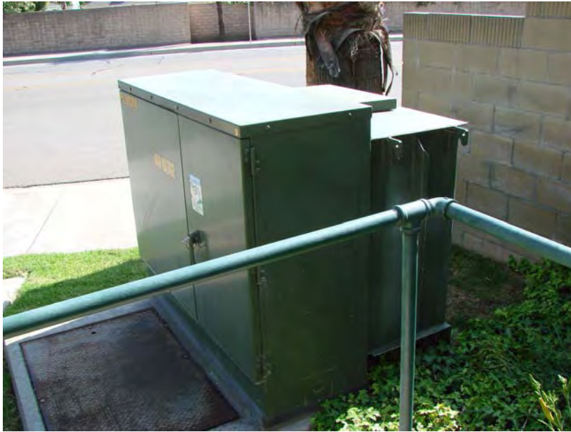
086 P_W: Pad mounted electrical transformer.
