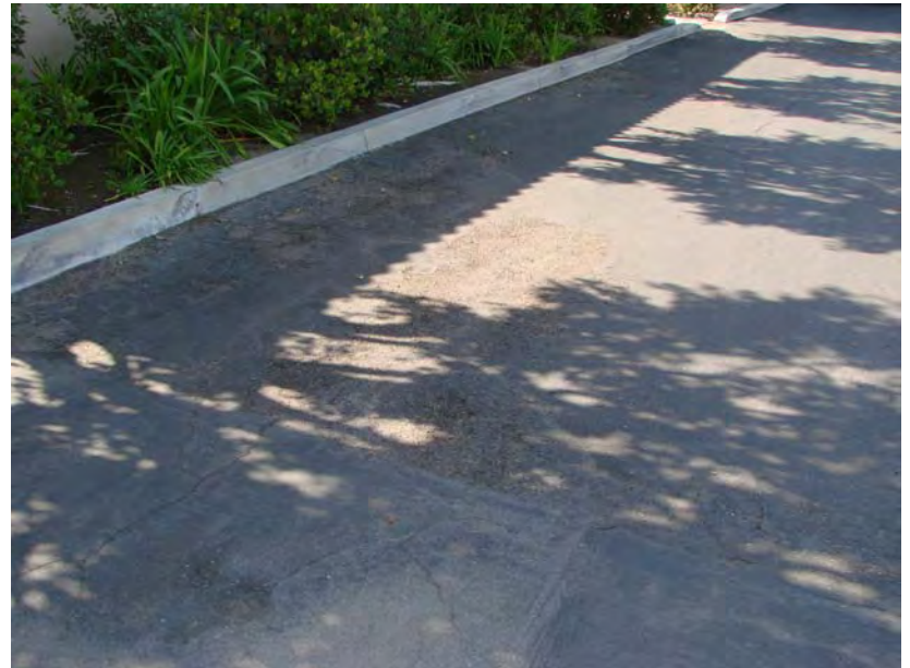
073 P_W: Paving detail - minor surface damage.
