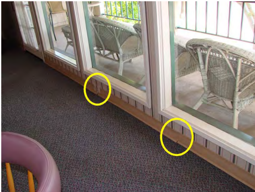
048 P_W: Detail - poor floor base installation.
