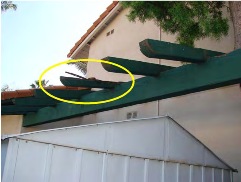
038 P_E: Detail - rotten beam.
