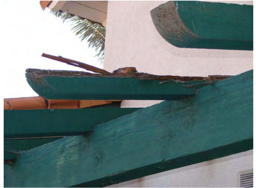
039 P_E: Detail - rotten beam.
