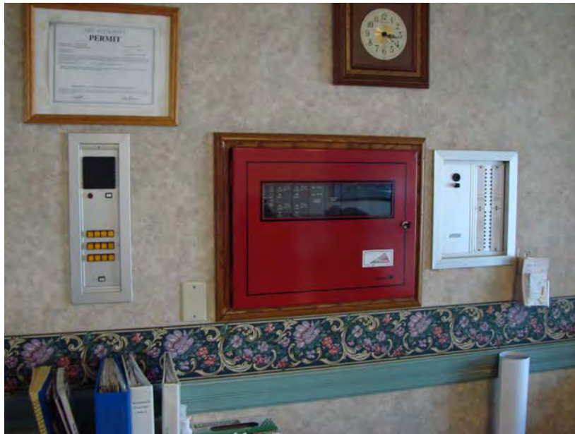
010 P_W: Palm West - Silent Knight fire alarm annunciator panel and Mirtone emergency-nurse call panel.
