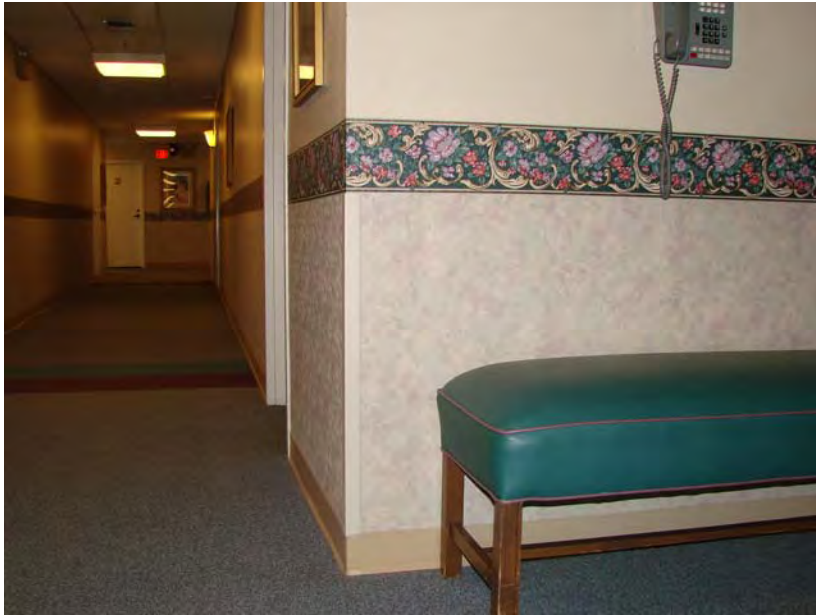
038 P_W: Corridor detail - carpet, rubber base, corner guards, wall covering below border, paint above border to ceiling.
