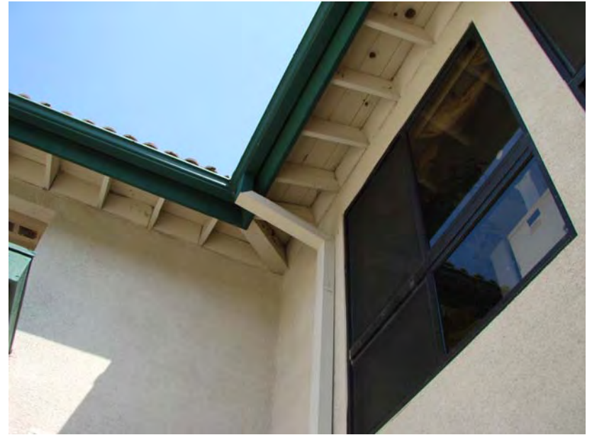
163 P_E: Detail - gutter, wasp nest under soffit.
