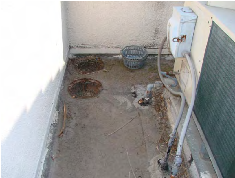
056 P_W: Roof drain in roof well - note drain covers out of place.
