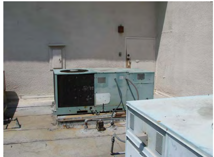
153 P_E: Rooftop HVAC unit - AC & gas heat.
