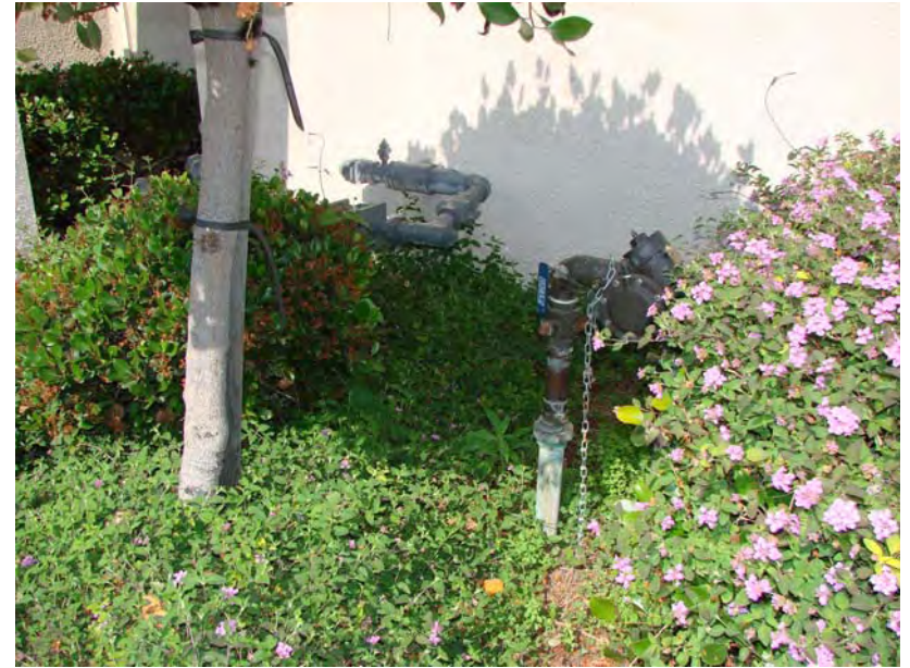
019 P_E: Irrigation sprinkler supply and gas meter.
