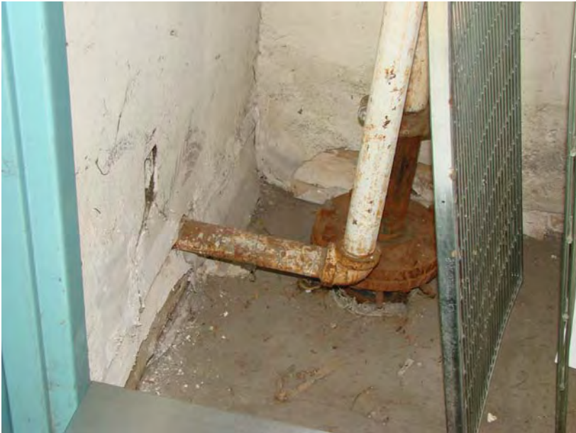
032 P_E: Water damage in water heater closet.
