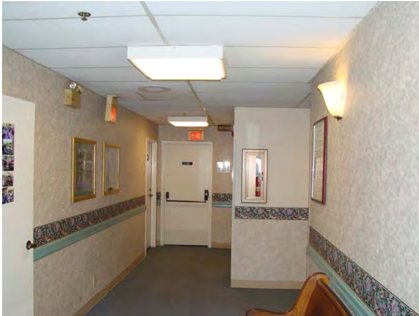
034 P_W: West end of South Hall; elevator. Note batter backup emergency light. Also note carpet, rubber wall base, wall paper, chair rail at handrail height,
