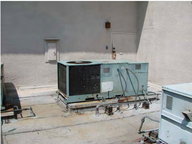
152 P_E: Rooftop HVAC unit - AC & gas heat.
