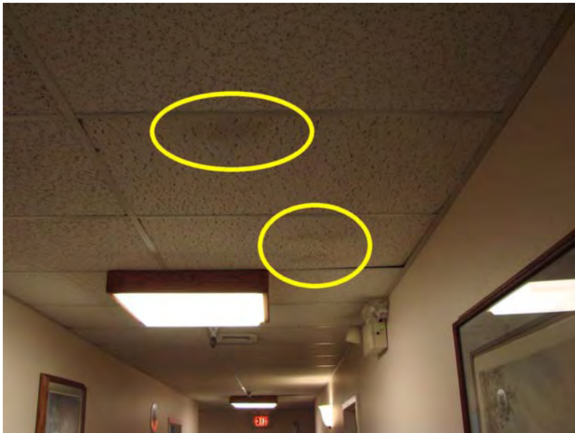
088 P_E: Darks spots on ceiling tile - consider repainting grid and replacing-painting ceiling tile.
