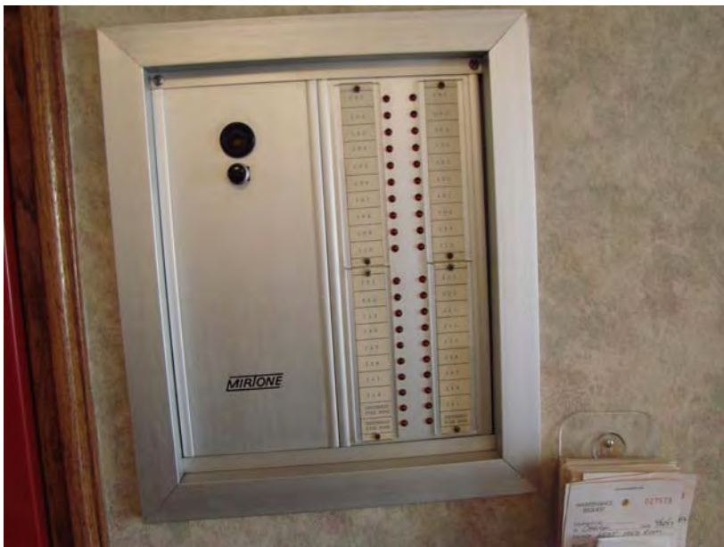
012 P_W: Mirtone emergency call system annunciator panel.
