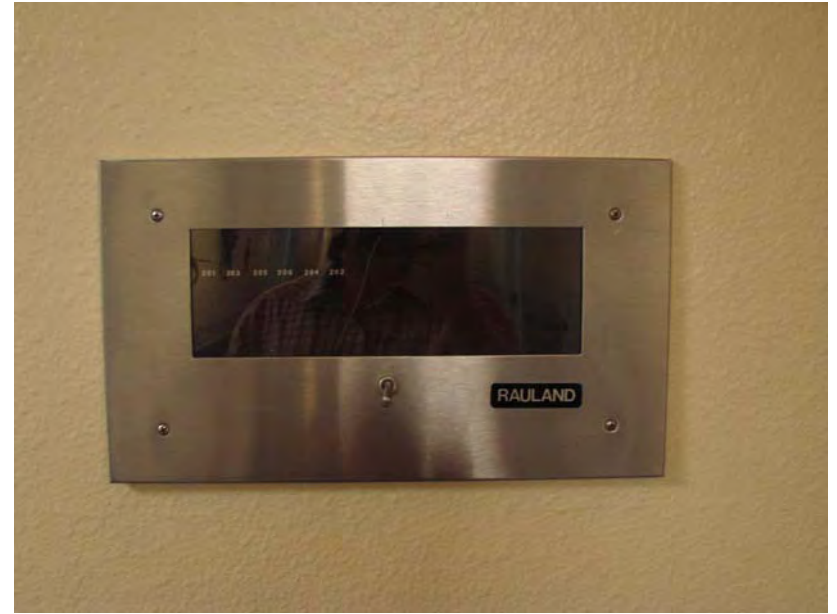
115 P_E: Rauland emergency-nurse call annunciator panel - 2nd floor (South end of West Hall).
