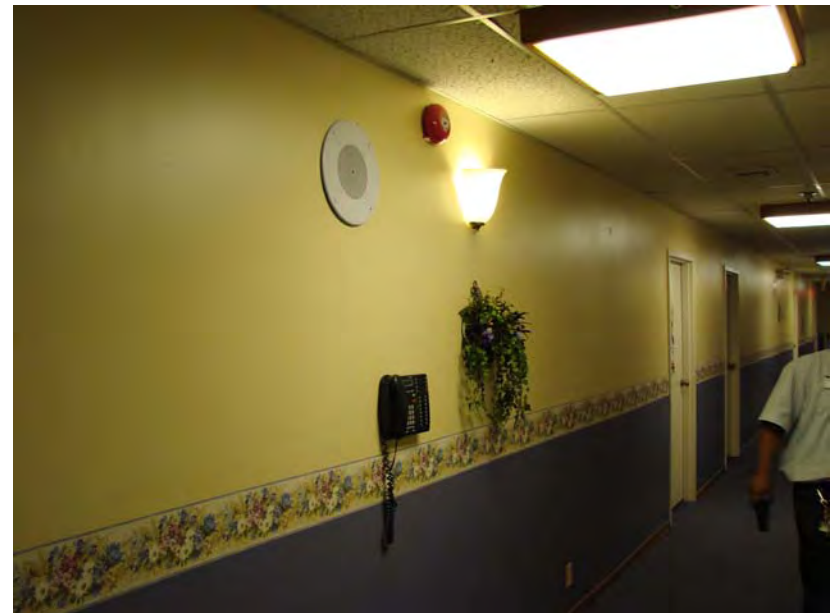
117 P_E: Public Address speaker, fire alarm, house phone - 2nd floor West Hall.
