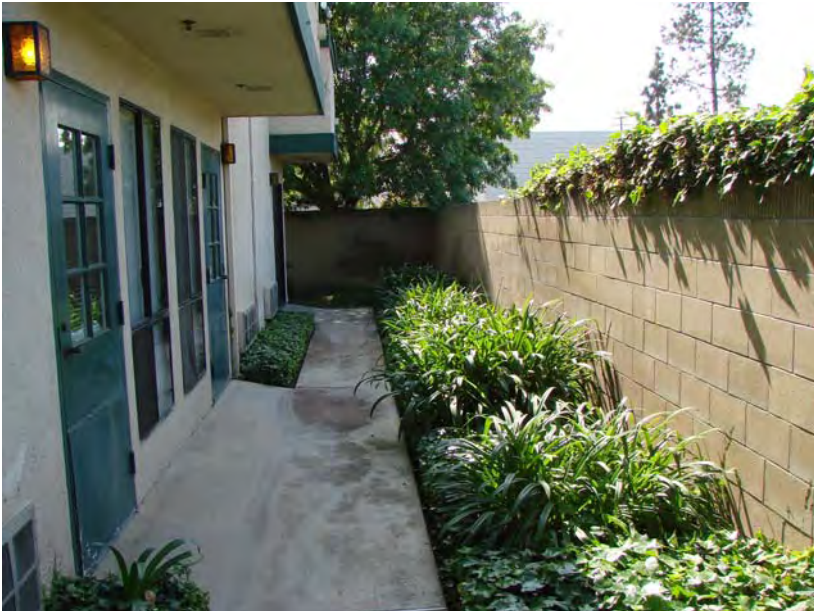
076 P_W: Sidewalk detail - slopes away from building, appears to pond some water.
