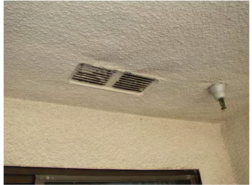
175 P_E: Soffit vent - needs to be cleaned.
