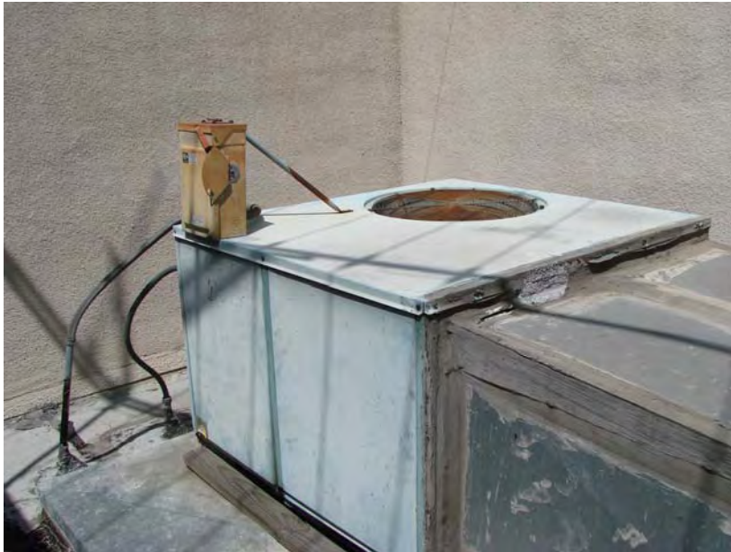
122 P_E: HVAC (AC & gas heat) unit in roof well above storage closet.
