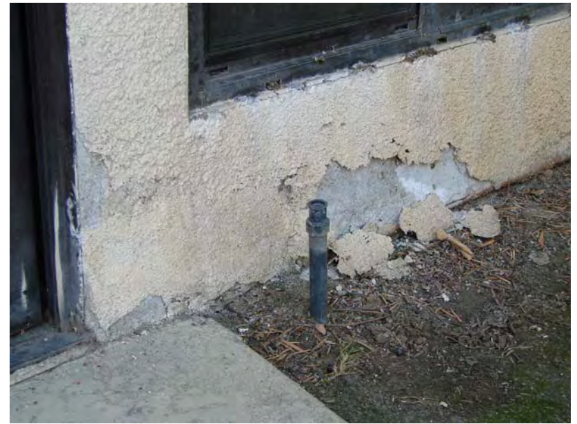
171 P_E: Water damage detail.
