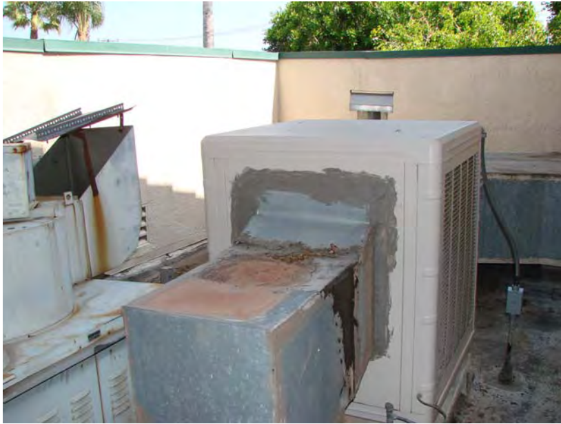
054 P_W: Kitchen swamp cooler in roof well.
