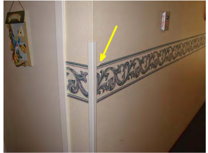
087 P_E: Detail - wallpaper border peeling at wall corner. (Note - staff has not yet begun 1st floor painting improvements.
