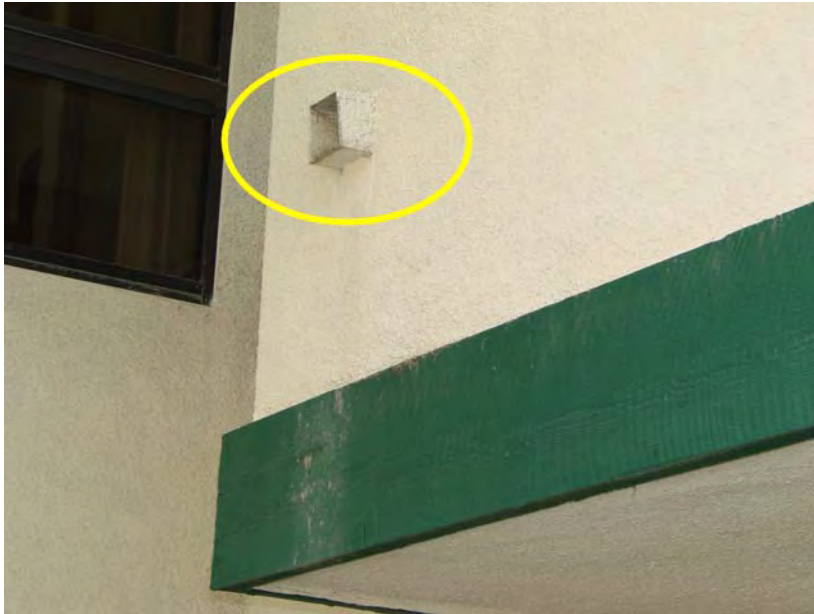
178 P_E: Detail - balcony drain. Consider adding drain scuppers to extend runoff beyond balcony wall.
