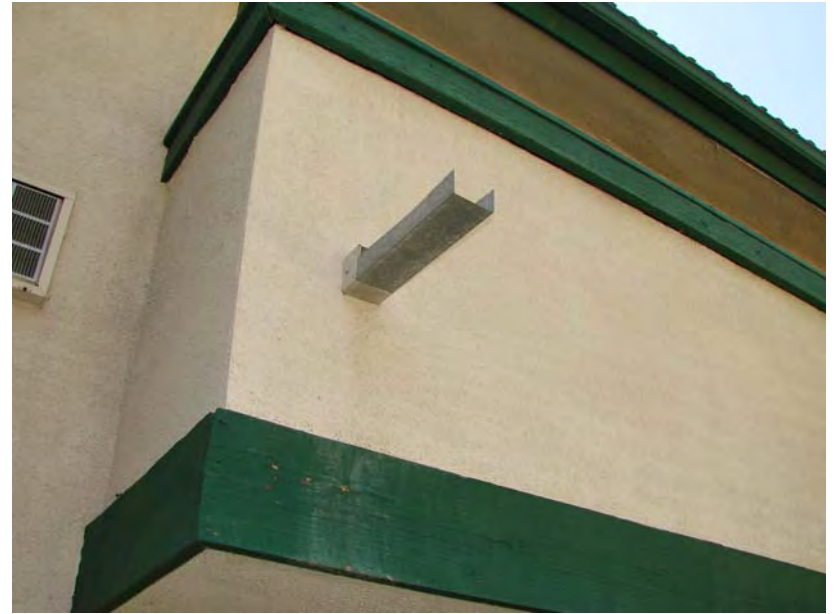
179 P_E: Balcony drain scupper with extension.
