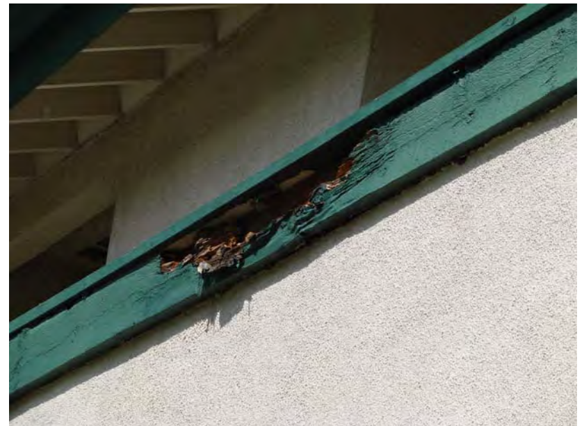
185 P_E: Detail - rotten wood trim on 2nd floor balconies.
