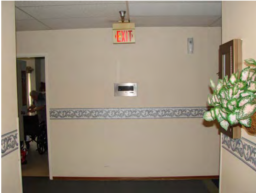
086 P_E: Rauland emergency-nurse call annunciator panel at north end of 1st Floor West Hall.
