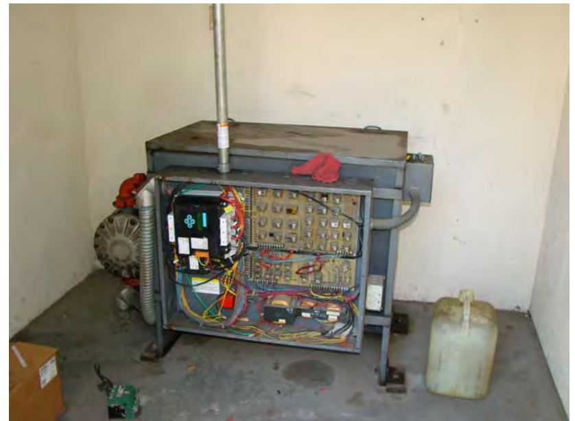
169 P_E: Hydraulic elevator equipment - recent repairs-maintenance.
