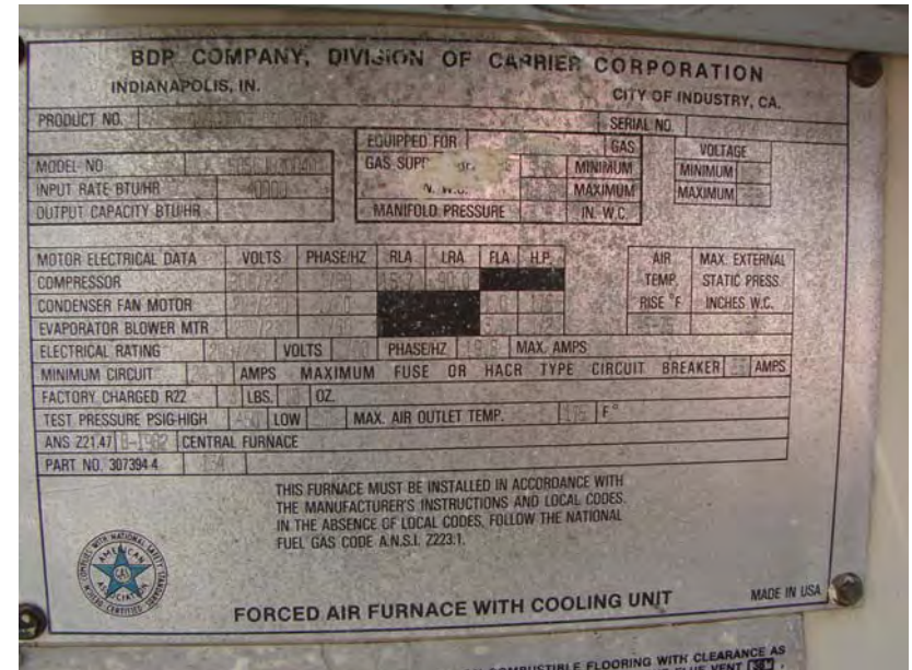
059 P_W: Day & Night HVAC unit in roof well - AC & gas heat.
