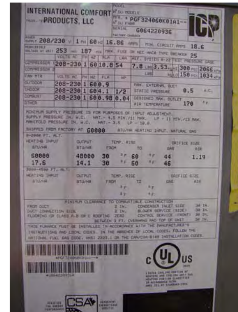
061 P_W: Heil HVAC unit in roof well - AC & gas heat.
