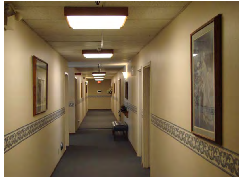
089 P_E: Typical 1st floor corridor - carpet, wood base, painted walls, wallpaper border at handrail height.
