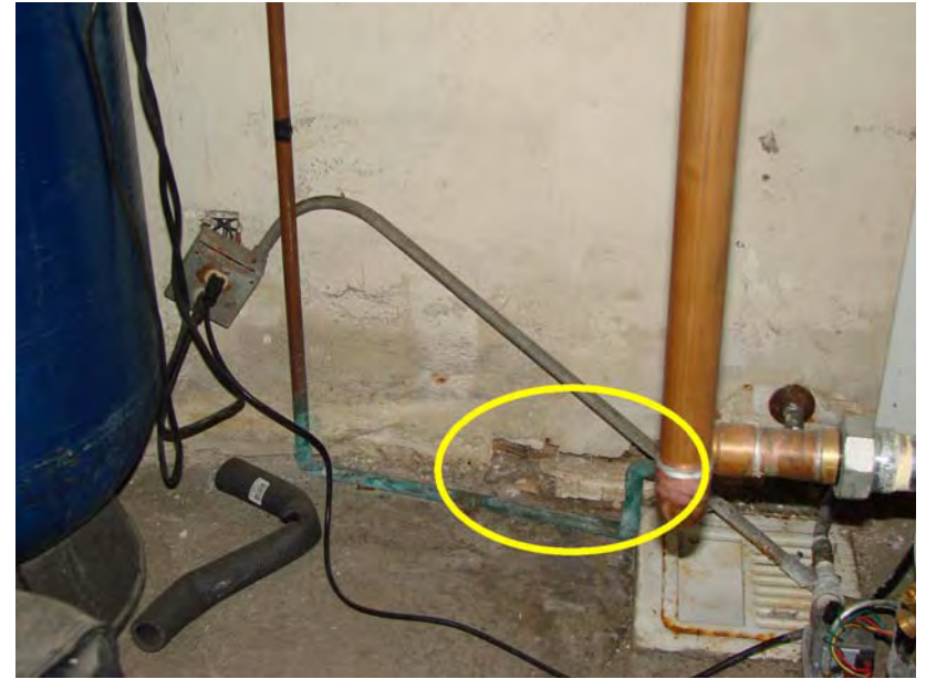
031 P_E: Water damage in water heater closet.
