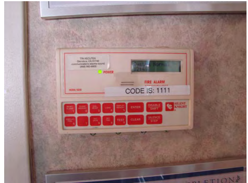
011 P_W: Silent Knight fire alarm annunciator.
