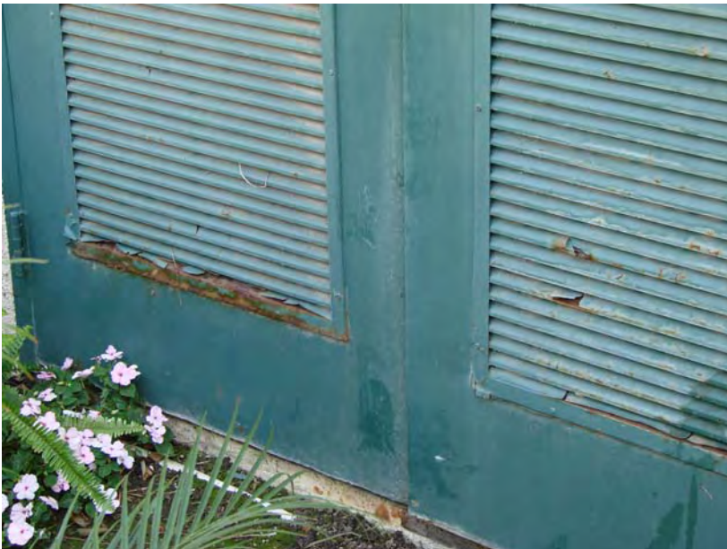
168 P_E: Detail of elevator equipment room doors - doors will need to be replaced in future years.
