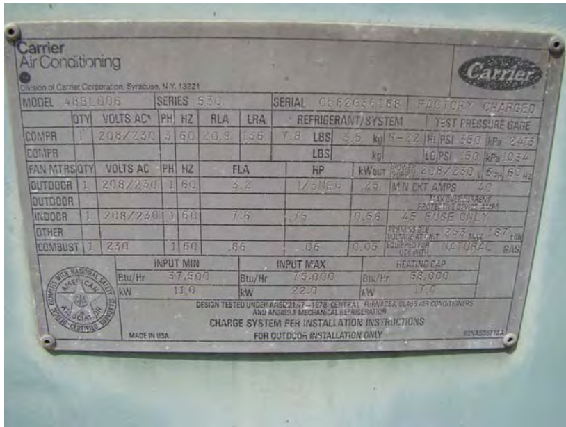
154 P_E: Rooftop HVAC unit - AC & gas heat.
